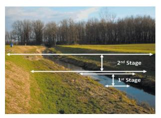
Two-stage ditches, like this one, create mini-floodplains within the channel.
