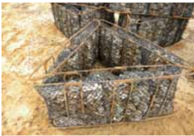
One of three oyster restoration projects in Alabama, ReefBLK cages are being used in Mobile Bay to create 750 linear meters of breakwater reefs. © Jeff DeQuattro/TNC
