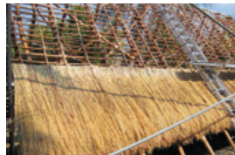
Partially completed hālau.
