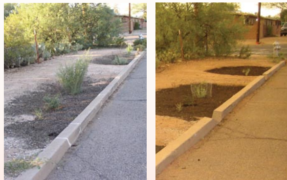
Cherry Ave. basins before and after curb cuts. Street runoff irrigates native trees, providing shade for pedestrians and habitat.
