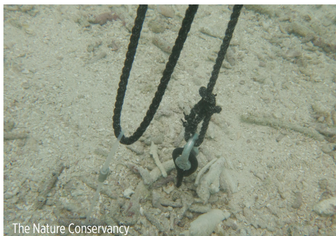
Figure 30. Examples of redundant anchor attachment methods; the first shows two anchors with slack in one line, and the second shows two anchors with equal length lines.
