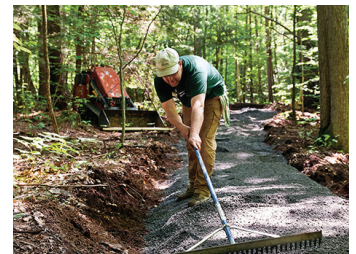
Trail work on the Boquet River Nature Preserve © Ken Aaron
