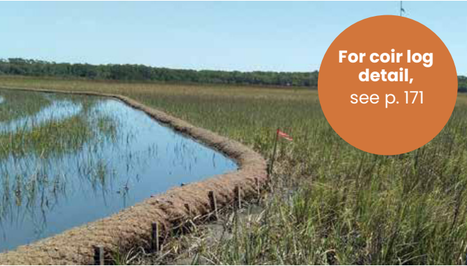
Coir Logs + Flexible + biodegradable - Limited height capacity
