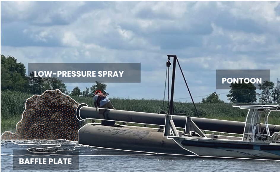
A pontoon-mounted pipe with a baffle plate directs low-discharge sediment slurry around a creek mouth, using controlled flow to minimize erosion and support natural sediment distribution.
