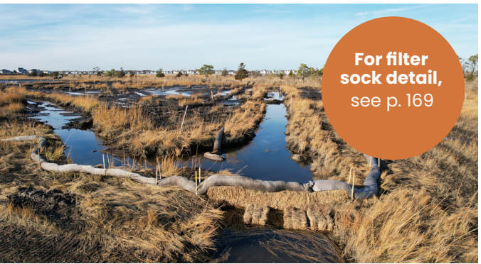
Filter Socks + Easy to install - Hard to remove
