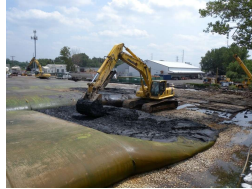
Dredging & capping contaminated soil
