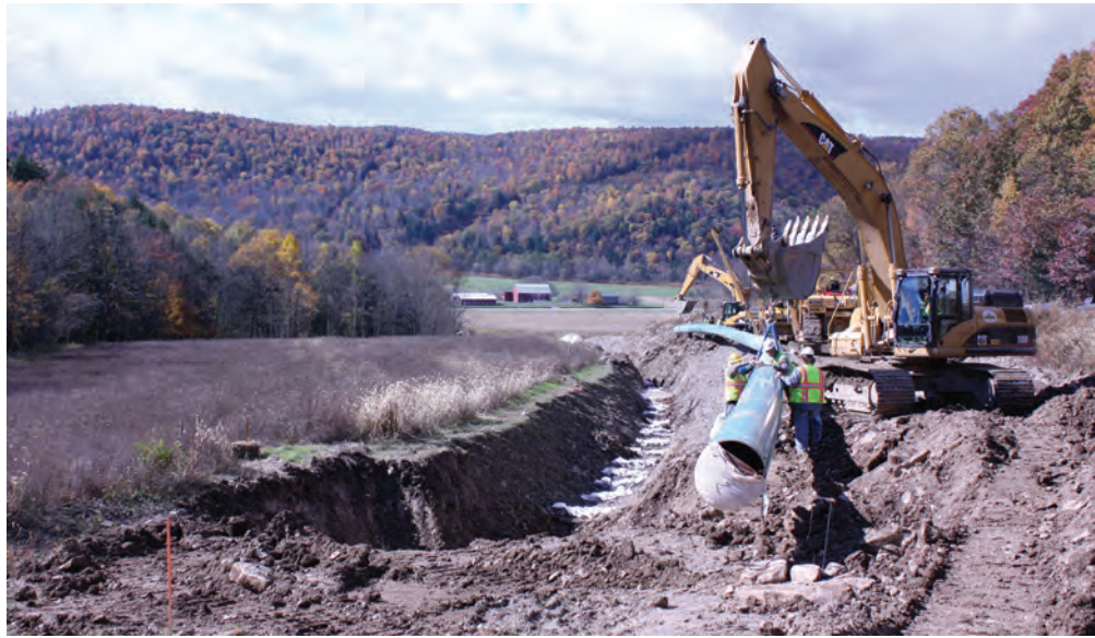
Clearing for well pads and pipes ©Cara Lee/TNC
