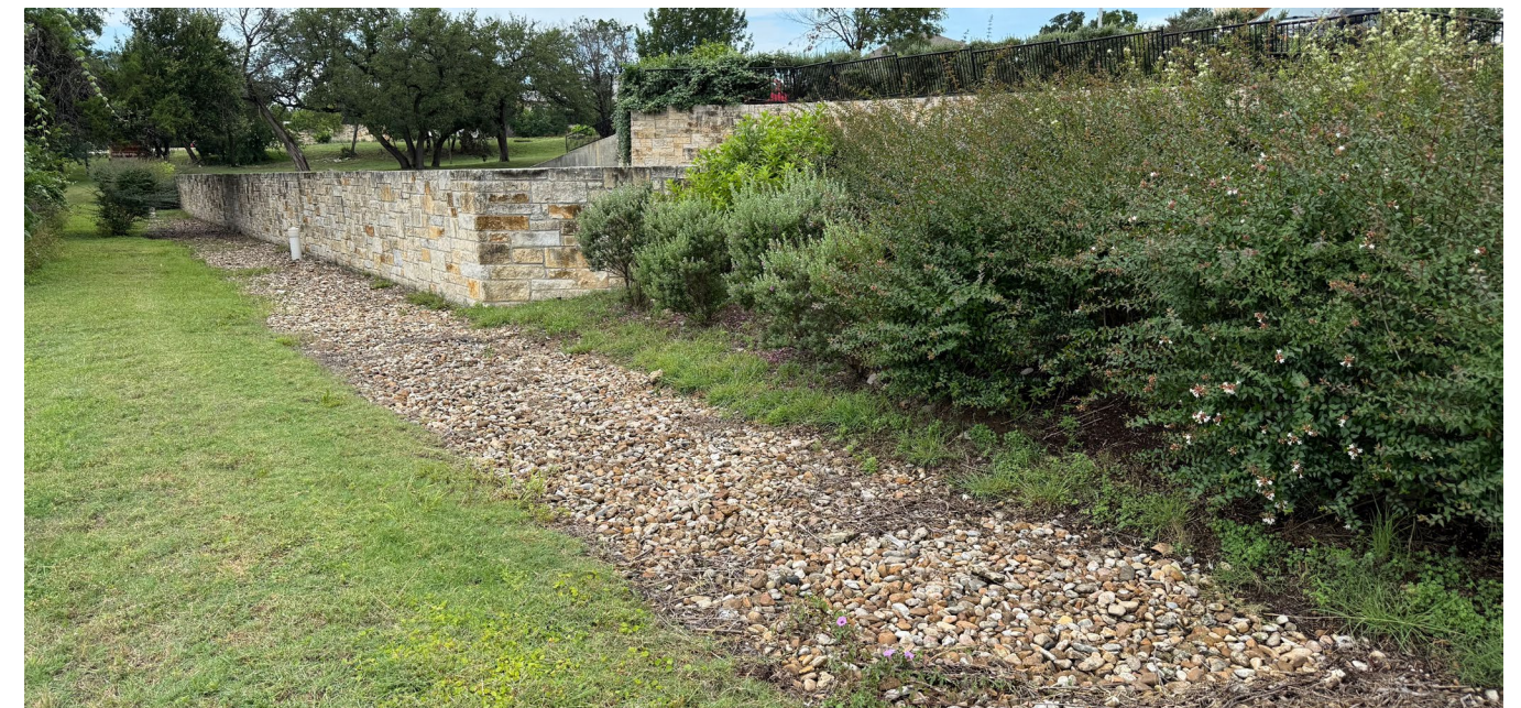
Figure 11-7. Infiltration Trench in Bee Cave, Texas
