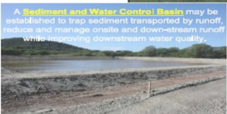
A Sediment and Water Control Basin may be established to trap sediment transported by runoff, reduce and manage onsite and down-stream runoff while improving downstream water quality.
