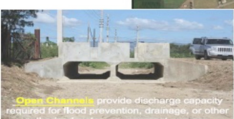
Open Channels provide discharge capacity required for flood prevention, drainage, or other authorized water management purpose.
