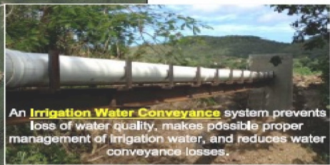
An Irrigation Water Conveyance system prevents loss of water quality, makes possible proper management of irrigation water, and reduces water conveyance losses.
