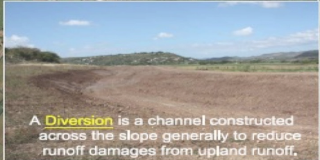
A Diversion is a channel constructed across the slope generally to reduce runoff damages from upland runoff.
