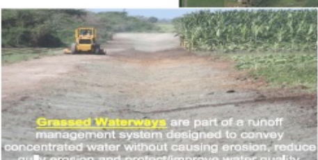
Grassed Waterways are part of a runoff management system designed to convey concentrated water without causing erosion, reduce gully erosion and protect/improve water quality.
