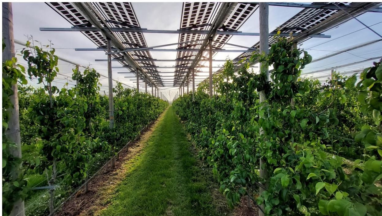
Figure 3. A pear agrivoltaic system in Europe. Image courtesy of Thomas Reher.
