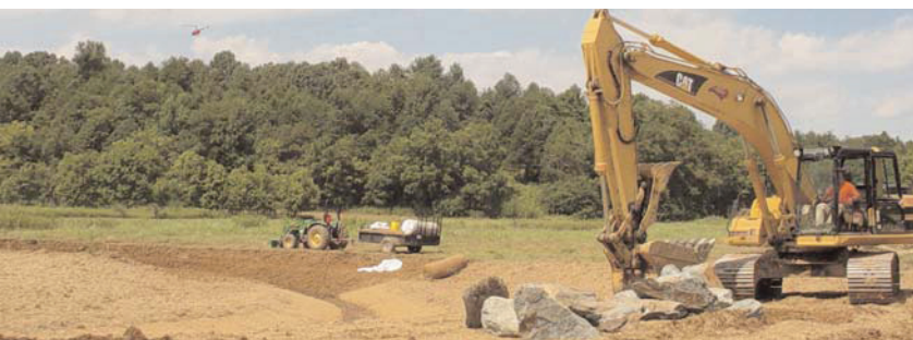
Crew from North State Environmental restores natural stream channel © Daniel White/TNC
