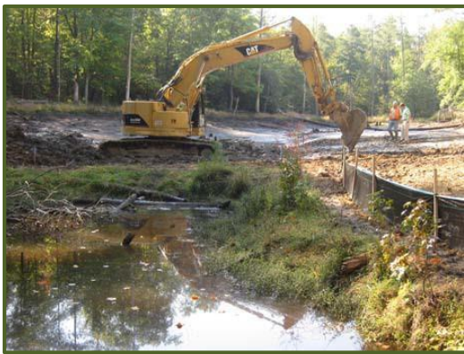
October 2010: Construction begins on the lower dam.
