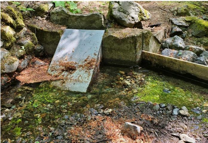
Figure 4. The current fish screen that will be replaced with a lower maintenance screen.
