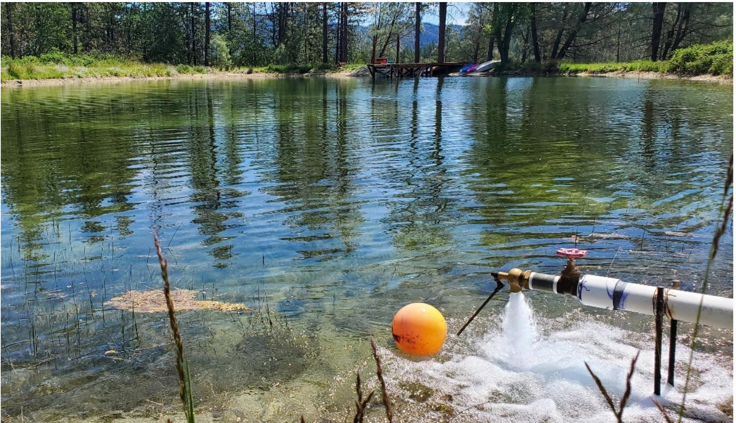
Figure 2. The trickle fill pond is being filled prior to the forbearance period. Note the orange ball attached to a float valve to stop the flow when the pond is full.
