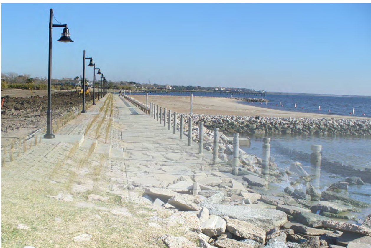
The Sylvan Beach project in La Porte, TX is a hybrid solution that created a community beach park using sand as a nature-based feature held in place by engineered rock groins.
