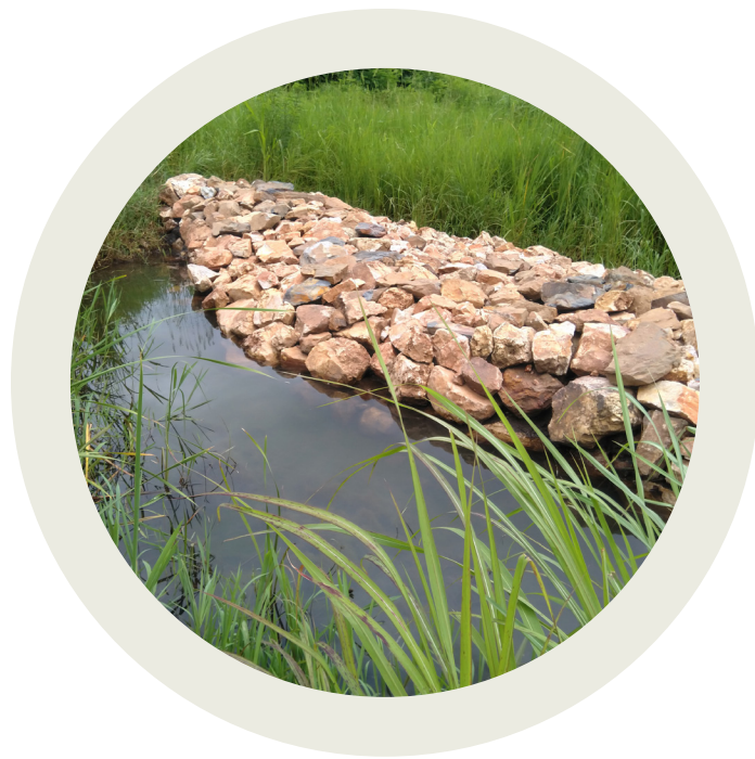
Leaky weir for enhanced water infiltration in the Kafue River catchment area, Zambia. © NIRAS
