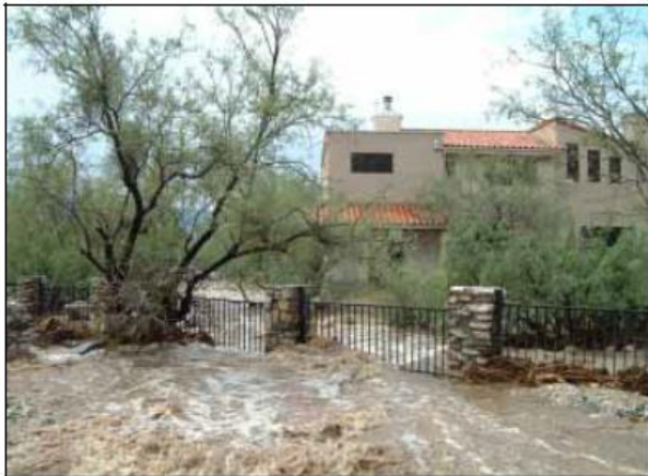
July 31, 2006, flooding event causing damage to nearby homes in Tucson, Arizona.
