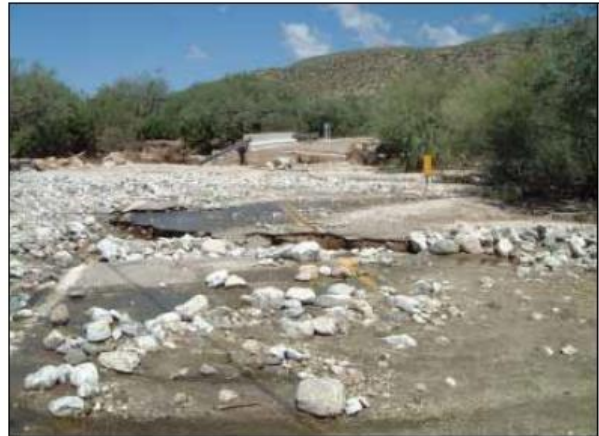
July 31, 2006, flooding event causing damage to roads and bridges in Tucson, Arizona.
