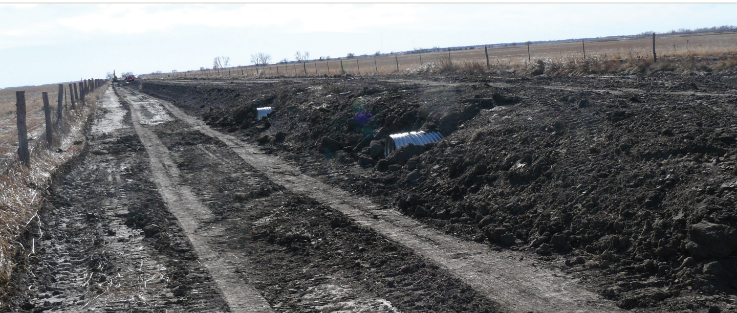
New culverts and a raised roadbed allow water to flow between the wetlands. © Robert Penner/TNC
