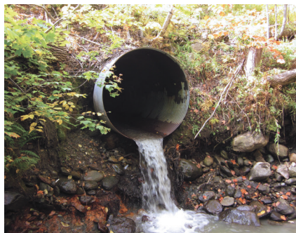
Stormwater Culvert © Sicker6/Creative Commons
