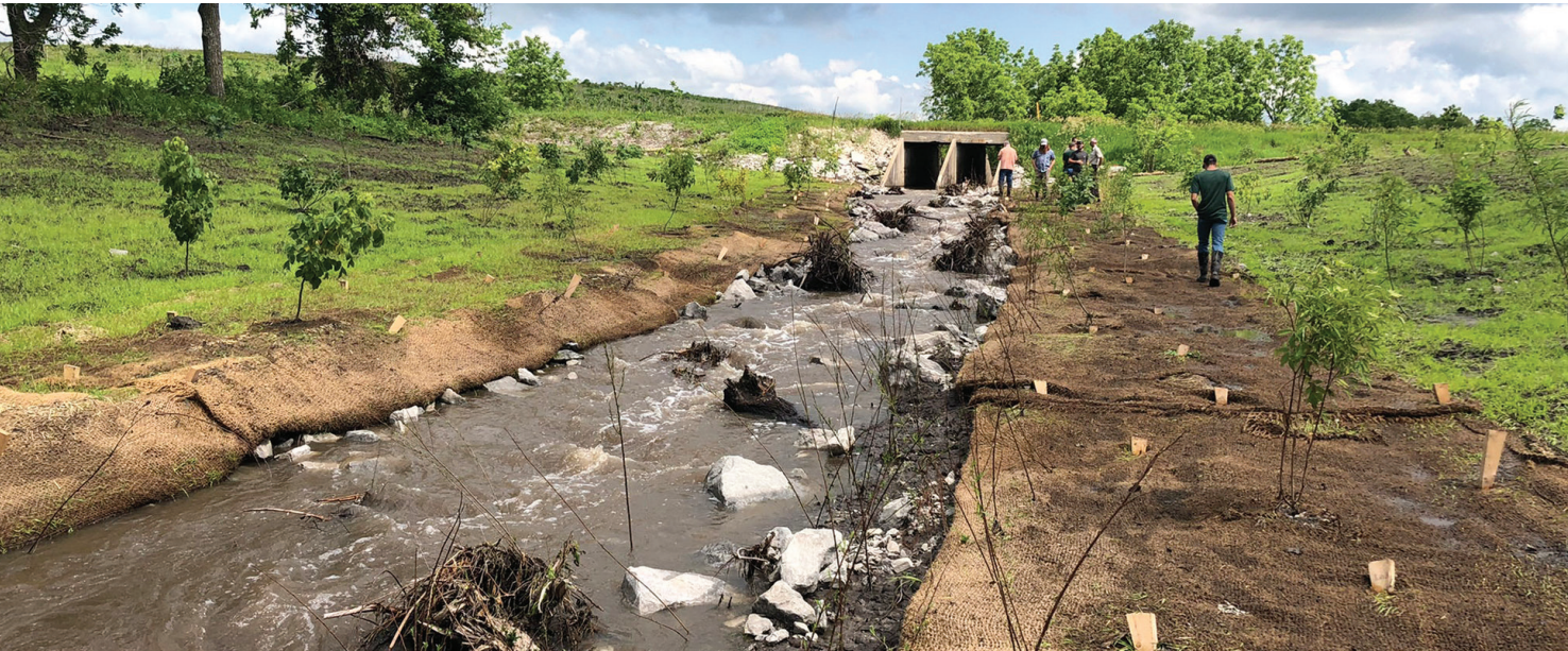
Little Creek's restoration is underway in Harrison County © Daniel Jensen/Shive-Hattery
