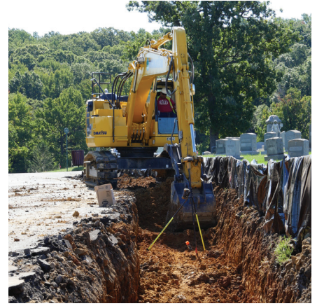
Impervious surface removal at Mount Olivet Cemetery, a project site where The Nature Conservancy is capturing stormwater runoff. © The Nature Conservancy
