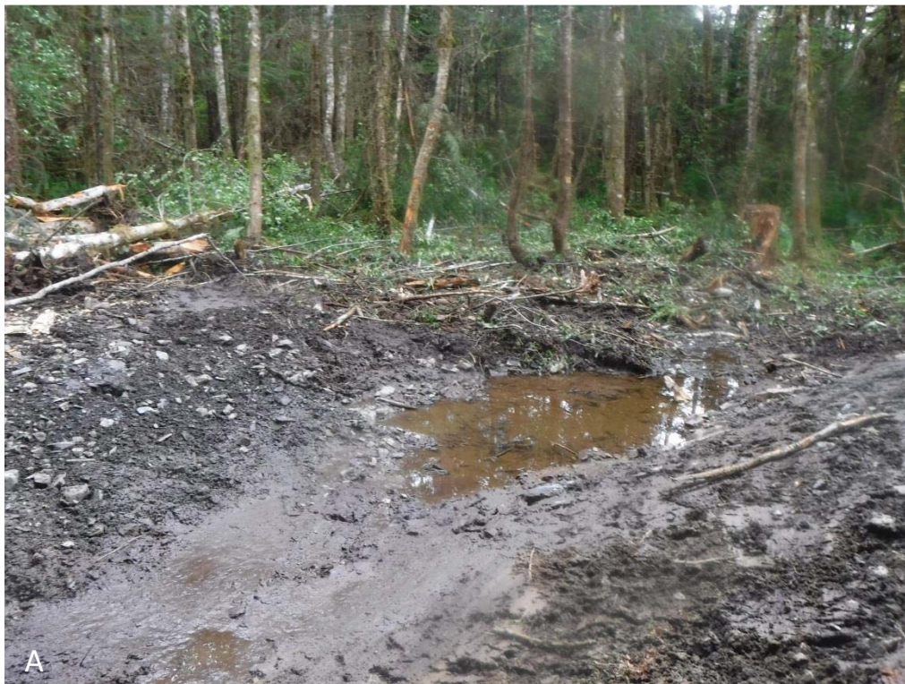
Figure 2. From the Pat Creek Fish Habitat Enhancement Project. (A) Example of a road breach excavated to the elevation of the surrounding grade on an alluvial fan. (B) Schematic of a typical road breach. (C) A logging road on an alluvial fan after removing alder trees to access breach sites.
