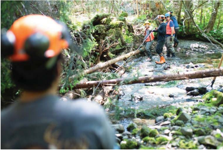
Figure 9. A large-wood structure constructed with hand tools in the Spaski Creek watershed on Hoonah Totem land on Chichagof Island. Photo by Ian Johnson.
