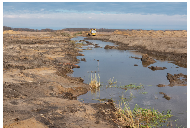
A bulldozer begins excavating the 12-acre wetland. ©Trevor Edmonson/TNC
