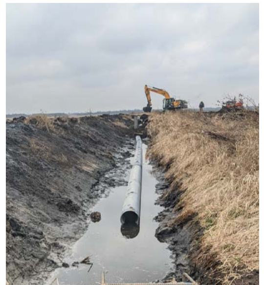
Ditch work being completed © Trevor Edmonson/TNC
