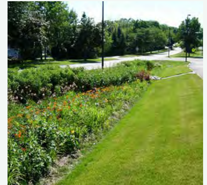
Bioswales are linear stormwater management systems that infiltrate, slow, and clean water when it rains
