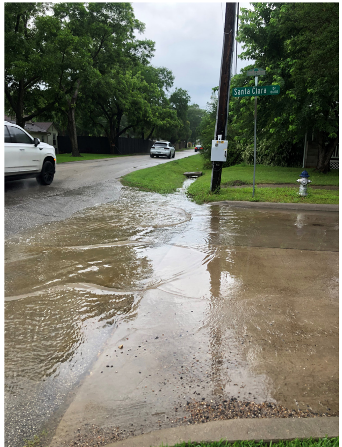
ABOVE: Inundated stormwater inlet. © Kathy Jack/ TNC
