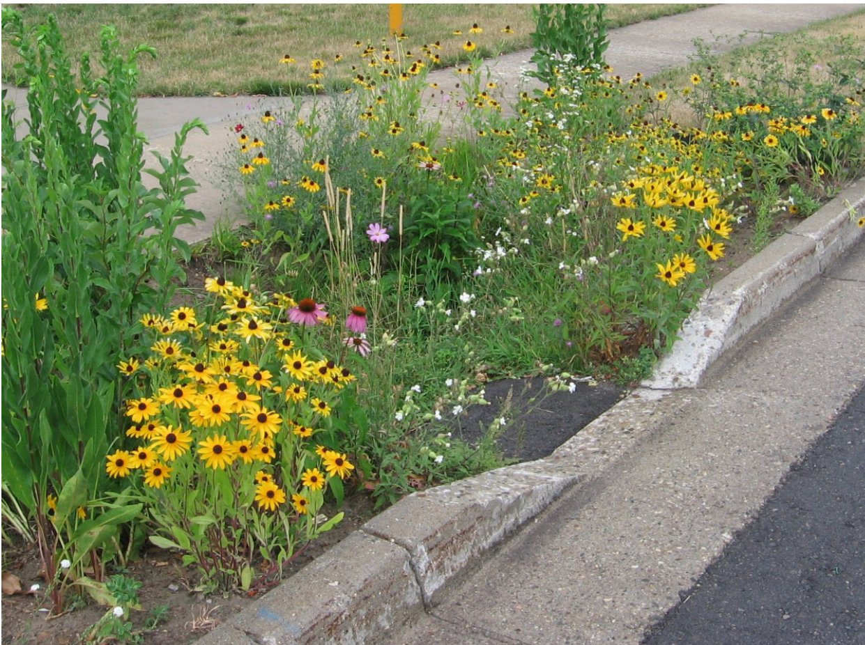
ABOVE: Rain garden with curb cut. © Texas A&M AgriLife
