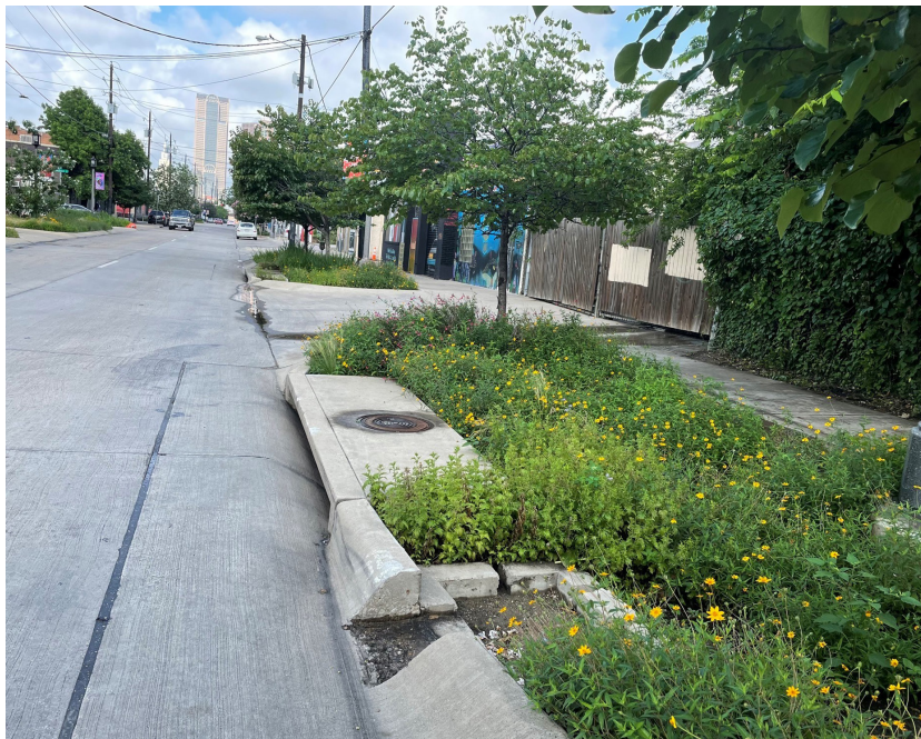
ABOVE: Sidewalk bioretention areas in Deep Ellum. © Katy Evans/ City of Dallas
