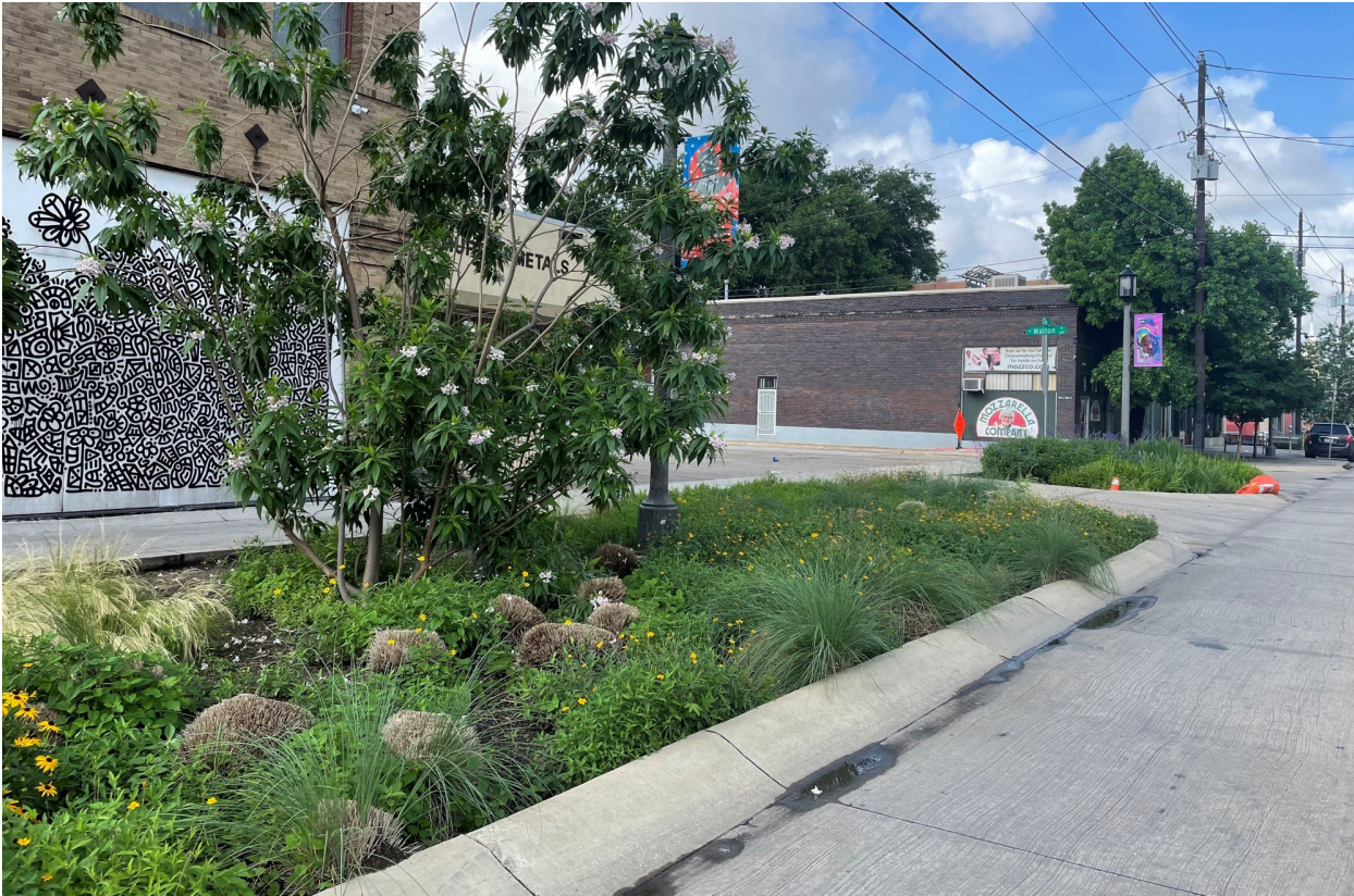
ABOVE: Sidewalk bioretention areas in Deep Ellum. © Katy Evans/ City of Dallas
