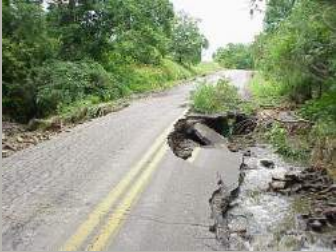
Road damage due to flooding. Photo courtesy of Steuben County Office of Emergency Services.
