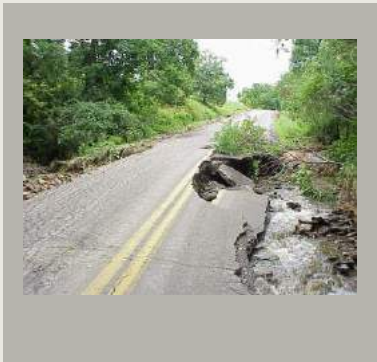
Road damage due to flash flooding and erosion, Steuben County. Photo courtesy of Steuben County Office of Emergency Services.
