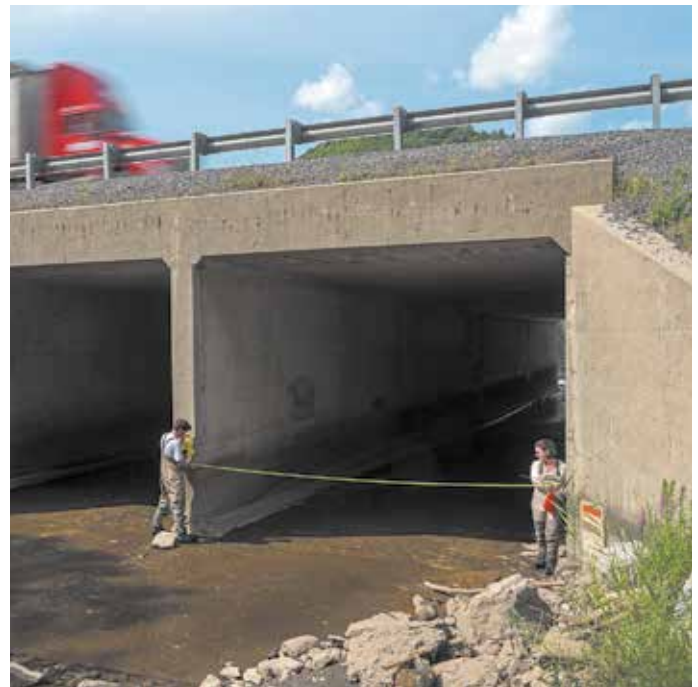
Field technicians perform an assessment along I-90. © John DiGiacomo
