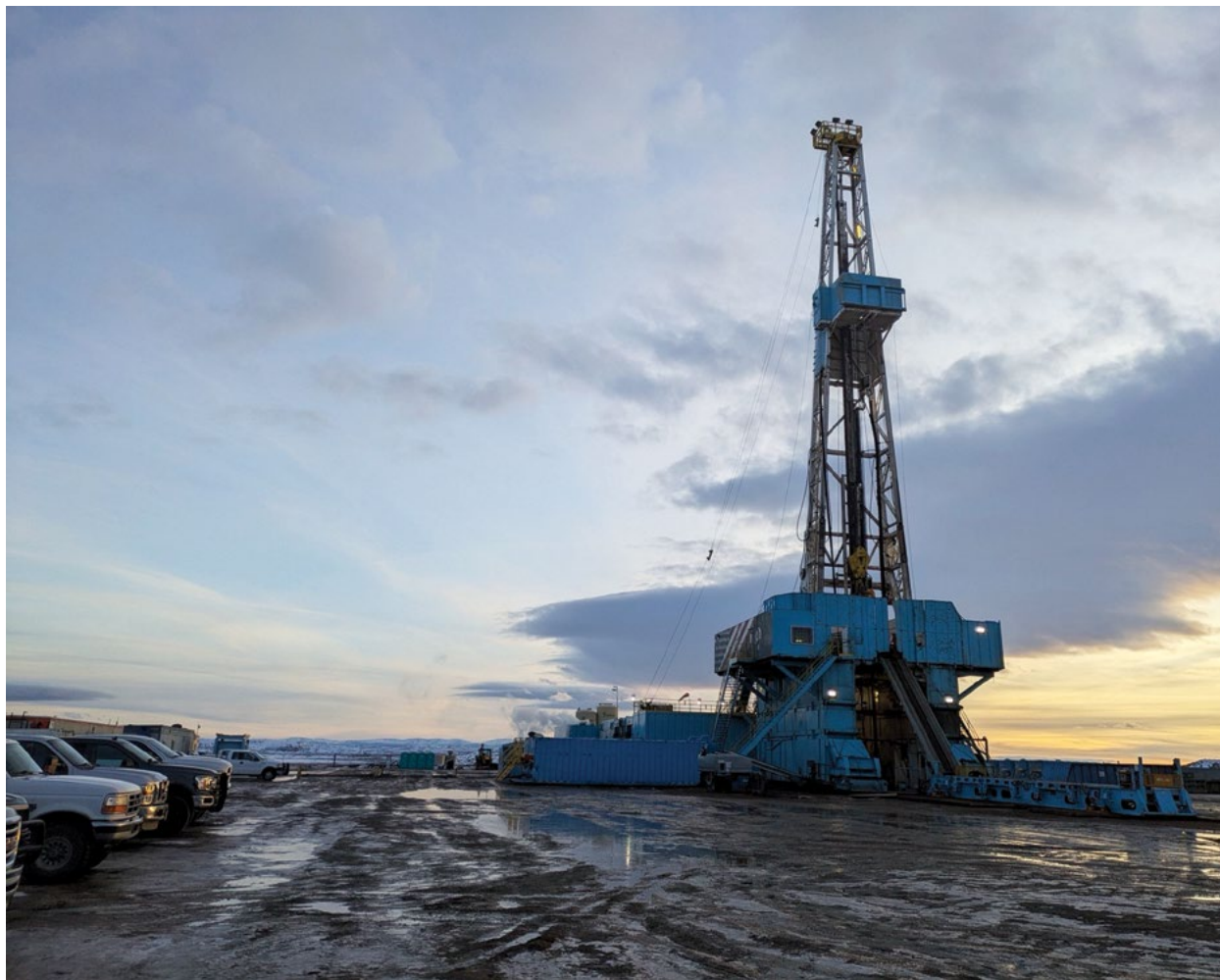
Wyoming's first Class VI well, drilled in Sweetwater County, specifically for the long-term geologic storage of carbon dioxide (CO 2 ) © Robby Rockey/Frontier Infrastructure, LLC
