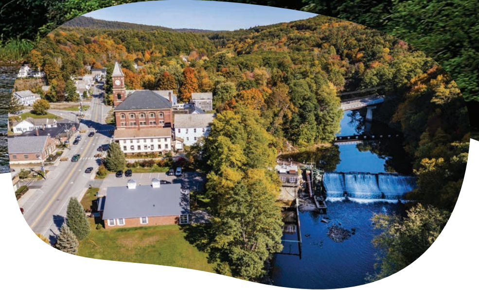
The Fiske Mill hydro dam on the Ashuelot River in Hinsdale, New Hampshire. © Jerry Monkman/ EcoPhotography.com
