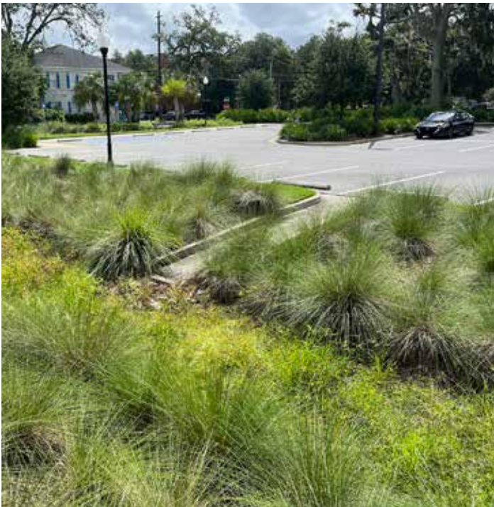
The city and local partners are implementing built green infrastructure practices to help soak up stormwater such as this large bioswale in the Veteran Memorial Park’s parking lot (left) or this permeable pavement at Liberty Ship Park (right).
