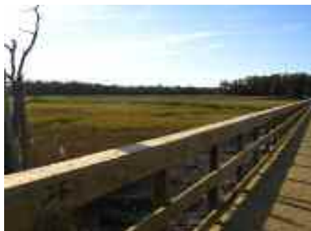
The new boardwalk at Eldora Nature Preserve © Dale Duffy Goldfarb
