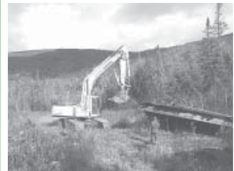
Removing bridges at TNC's Vickie Bunnell Preserve. Peter Benson photo © TNC.
