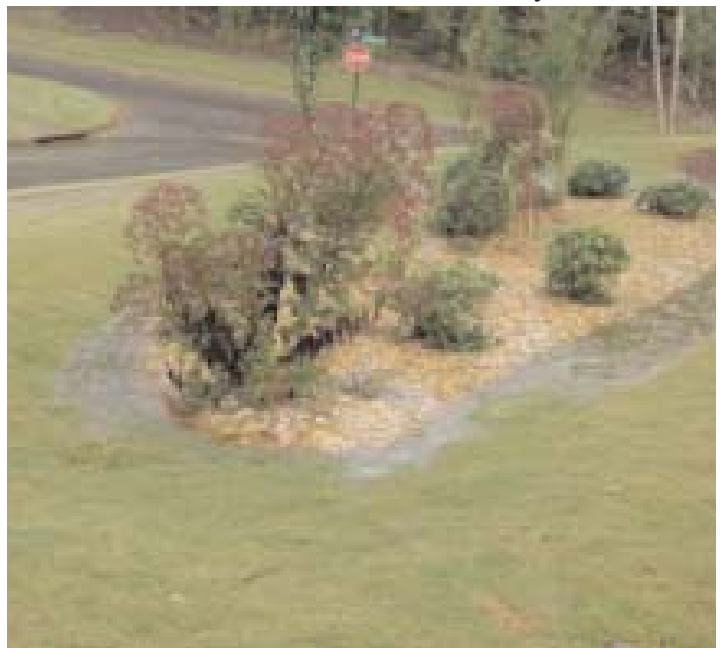
This rain garden in the Brooke Park subdivision in Canton absorbs stormwater runoff from a parking lot. © Candace Stoughton/TNC
