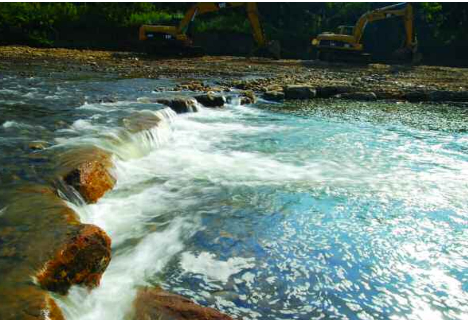
Shown above is one of the structures used to direct the energy of the Middle Fork of the Little Red River away from an eroding bank. © Ethan Inlander/TNC
