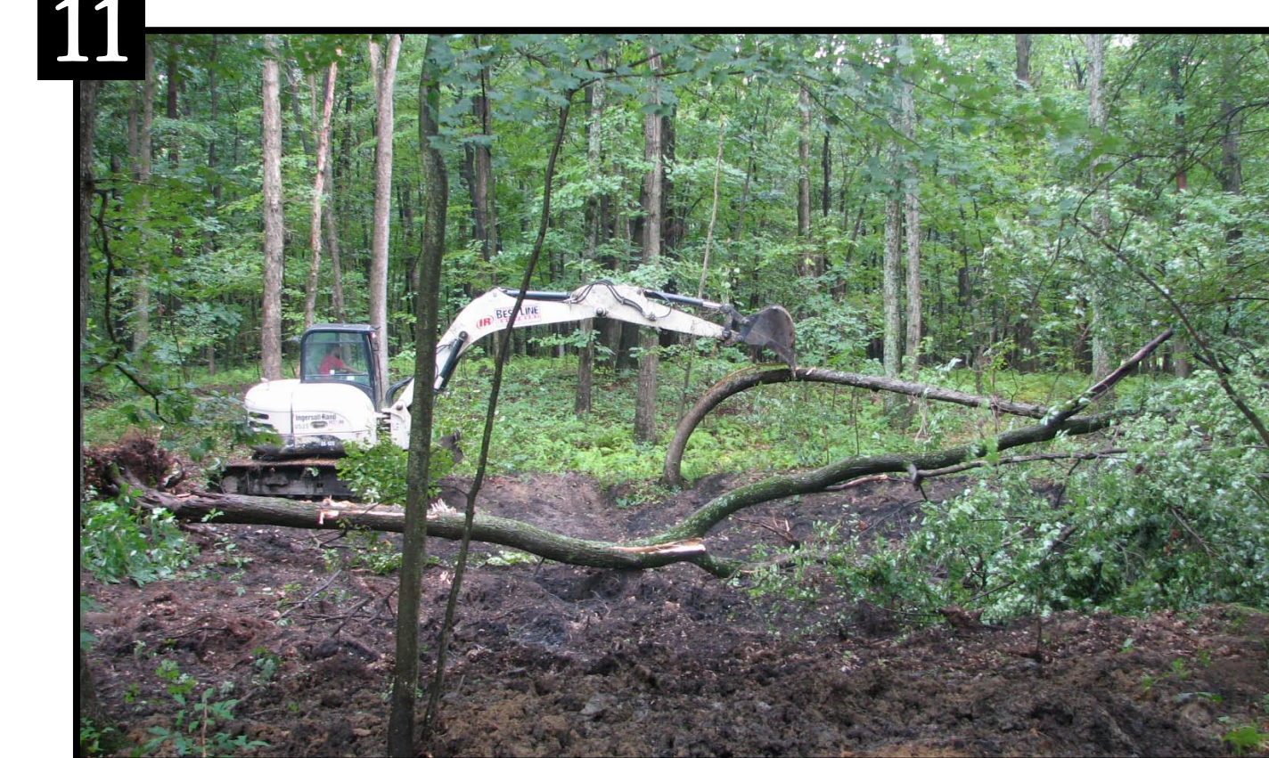
11 The excavator pushed two large trees and other woody debris into the completed wetland to provide habitat for salamanders and discourage the use of motorized vehicles within the wetland.
