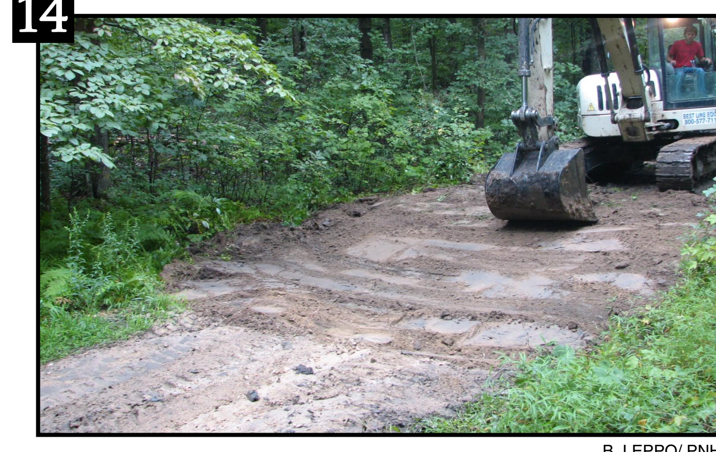
14 Water flowing down a grassy Right-Of-Way was directed into the pool by creating a shallow dip at the lowest point in the ROW upslope from the wetland.
