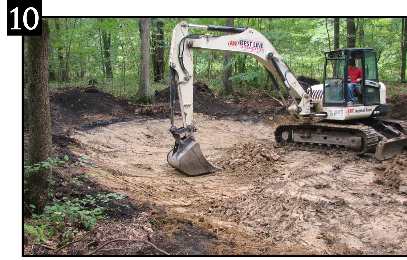
10 The loose clay soils were returned to the pool basin in 4-inch layers. Each layer was compacted with the bucket on the excavator.
