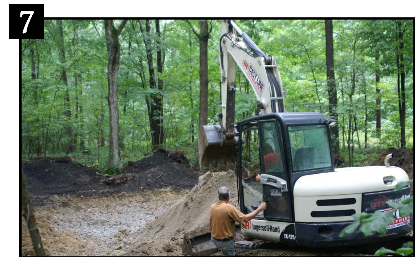
7 As in the liner and ground water techniques, the leaves and topsoil were removed and reserved. Twelve inches of sandy loam mineral soil were removed and taken to a restoration site on private property.
