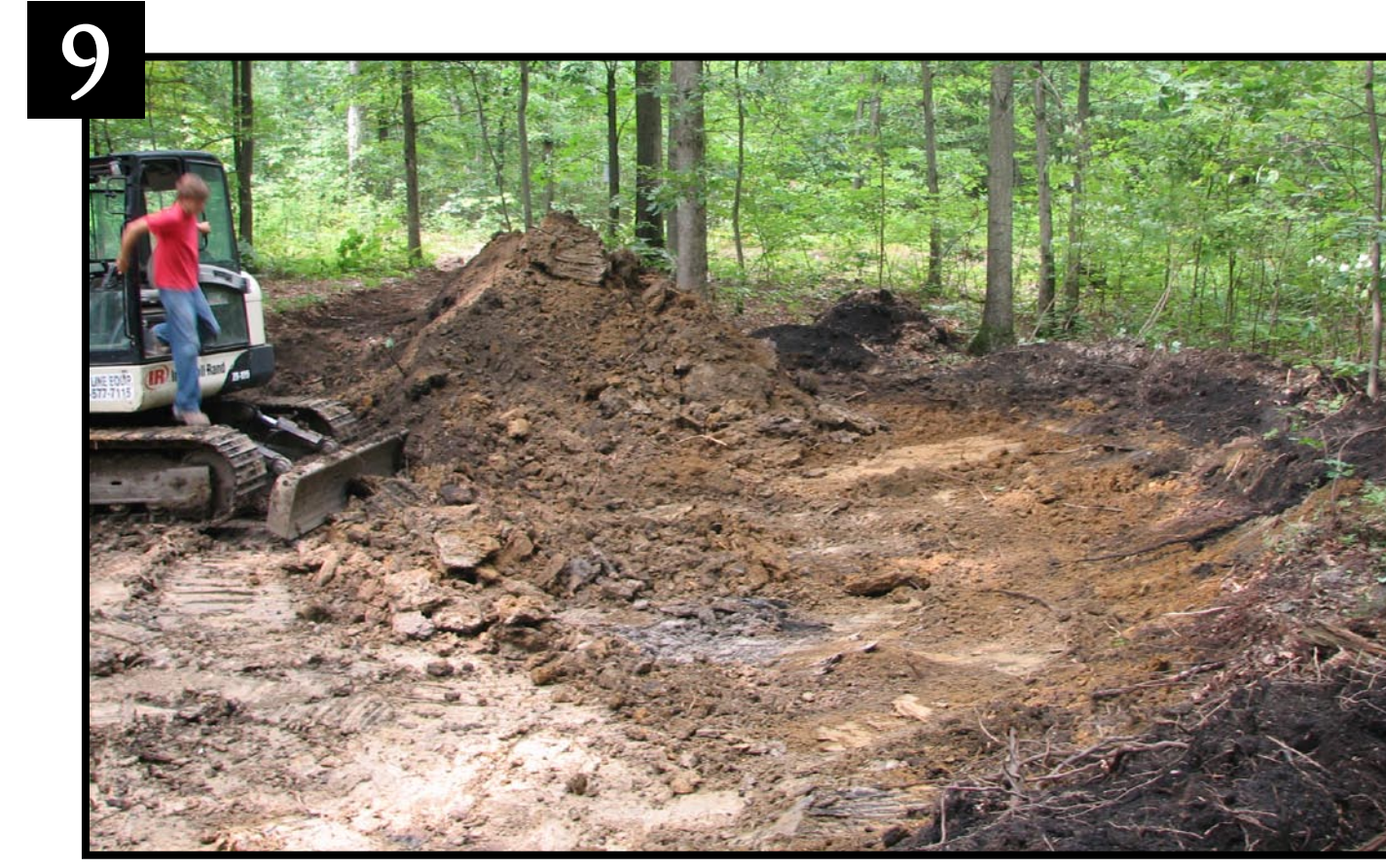
9 The sandy loam covered a layer of loose clay, which was removed to a depth of 3 feet and reserved. Compacted clay over sand and sandstone rock was found beneath the loose clay.
