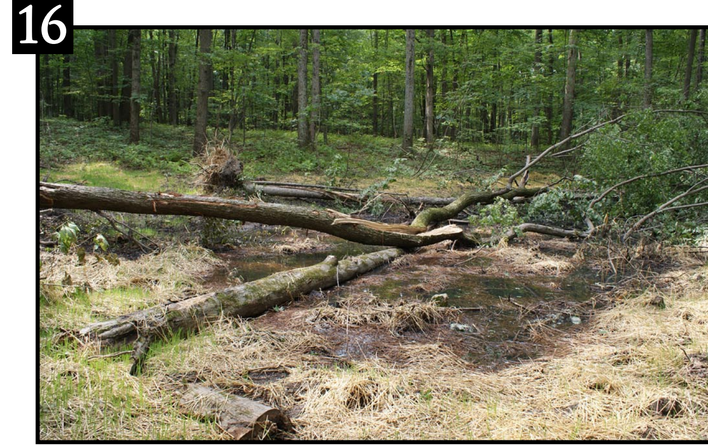
16 The completed basin is 60 feet in diameter and has an average depth of 17 inches.
