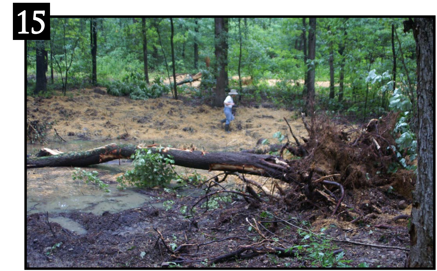
15 One day after construction, the wheat and straw provided erosion control during a steady rainfall. The newly compacted clay layer slows the rate at which water seeps into the ground.
