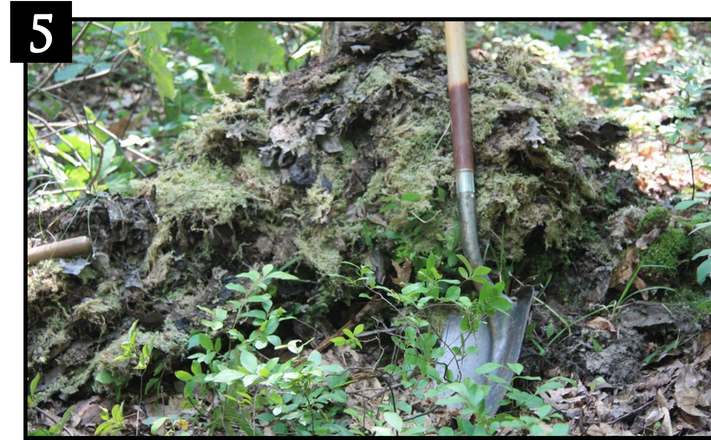
5 Prior to construction the vegetation, leaf litter, and topsoil were removed from the basin and reserved.
