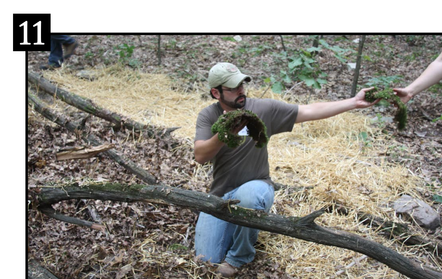
11 After returning leaf litter and plants to the basins, wheat or oat seed and clean straw were spread within the construction area to control erosion and deter invasive plants.
