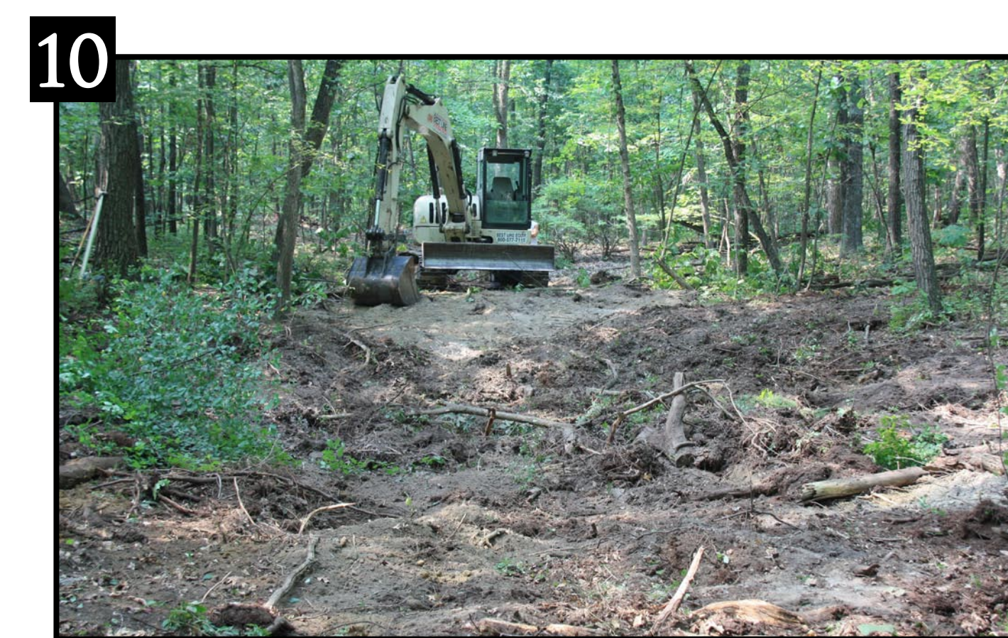
10 Once the basins were bowl shaped with gradually sloping sides, the excavator placed the reserved topsoil into the deepened basin.
