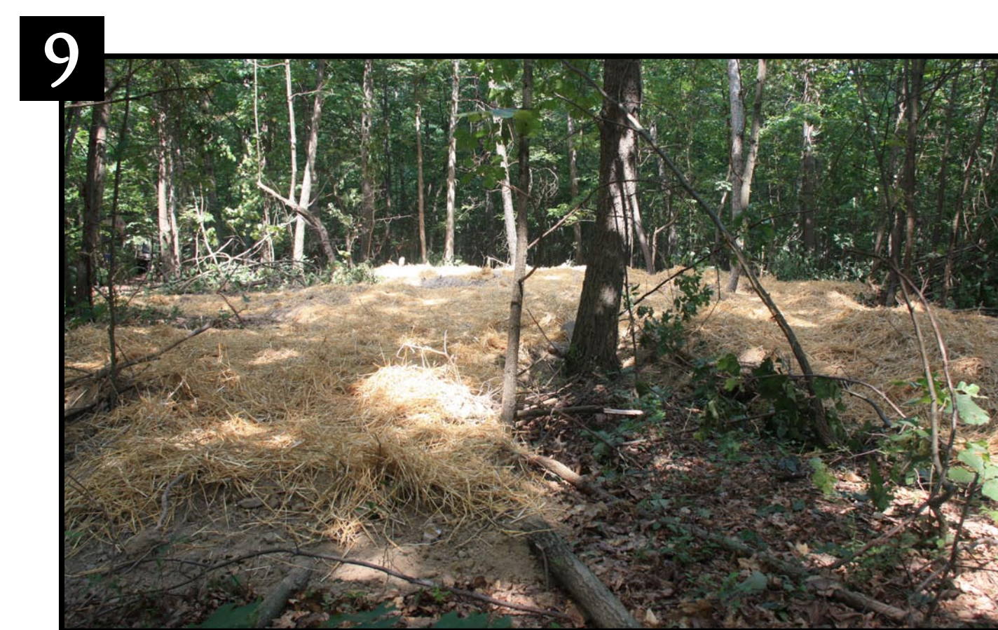
9 The excess soil location was seeded with wheat and covered with clean straw for erosion control.
