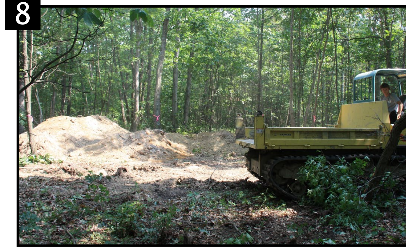
8 The excess mineral soil from each basin was spread (not compacted) in a nearby flat upland to avoid erosion into the deepened basin.
