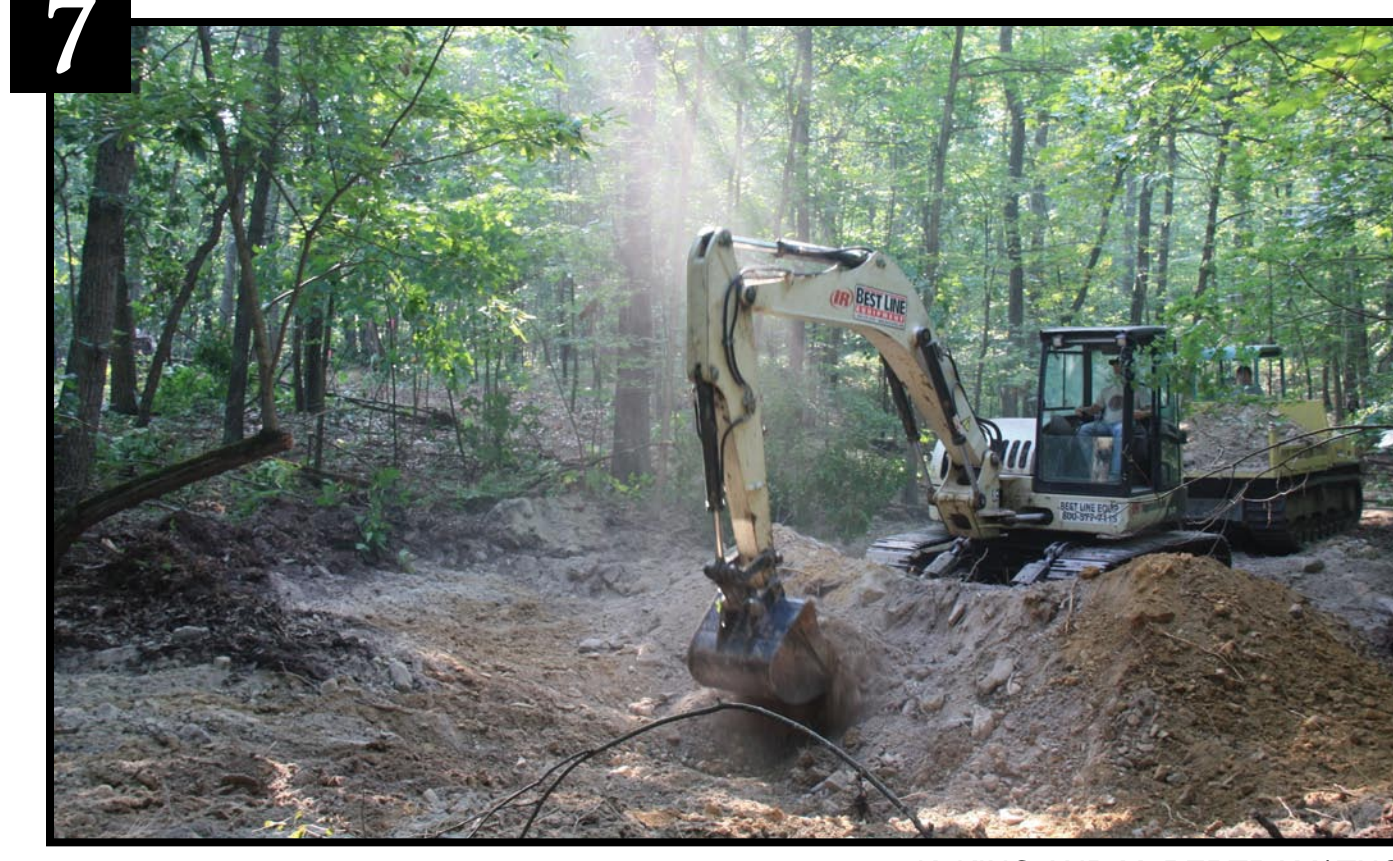
7 To lower the profile, an excavator with a 40 inch bucket removed 16-19 inches of mineral soil from each basin.
