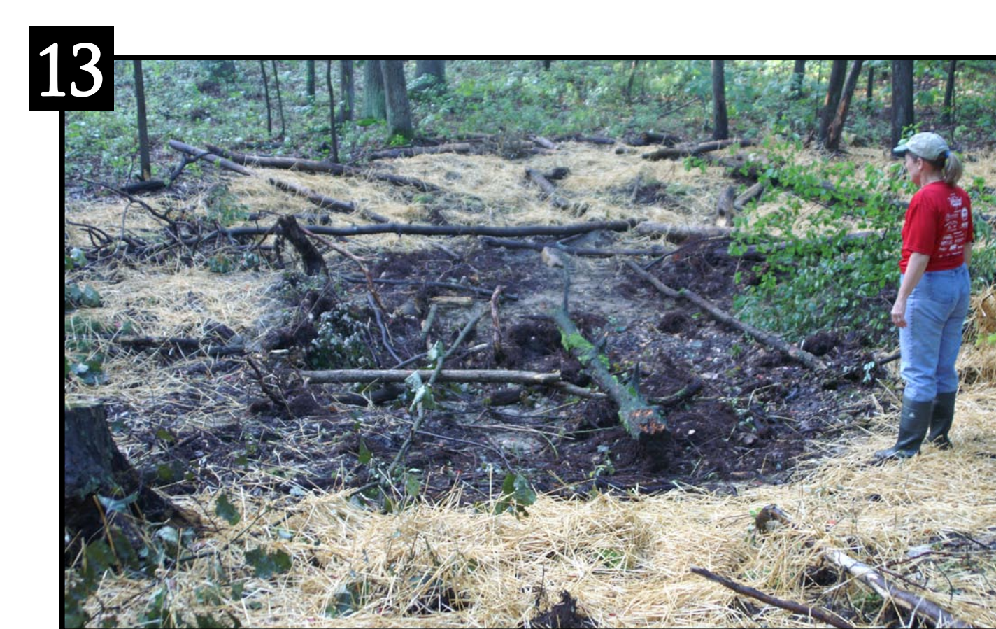
13 A few days after construction the wheat and straw provided erosion control during a steady rainfall.
