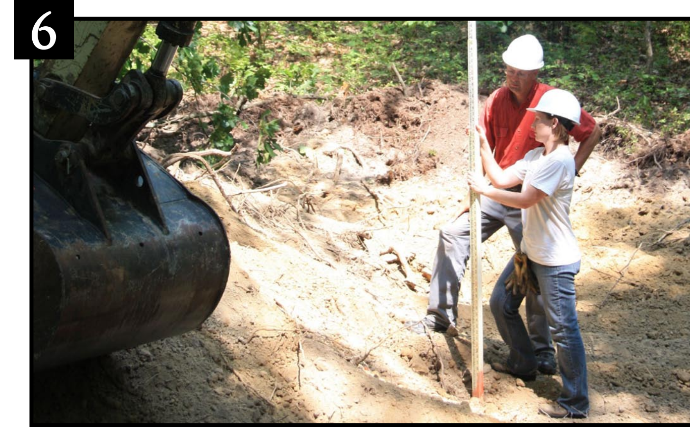
6 The dimensions of the pool basins were checked periodically to provide guidance to the equipment operators so that they could match the restoration design.
