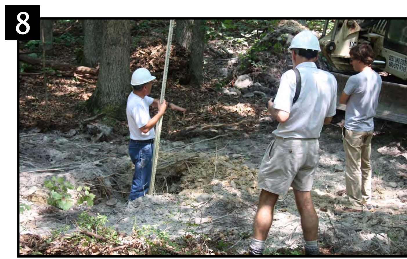
8 A test hole was dug by the excavator, and the target maximum depth measured with the construction level.
