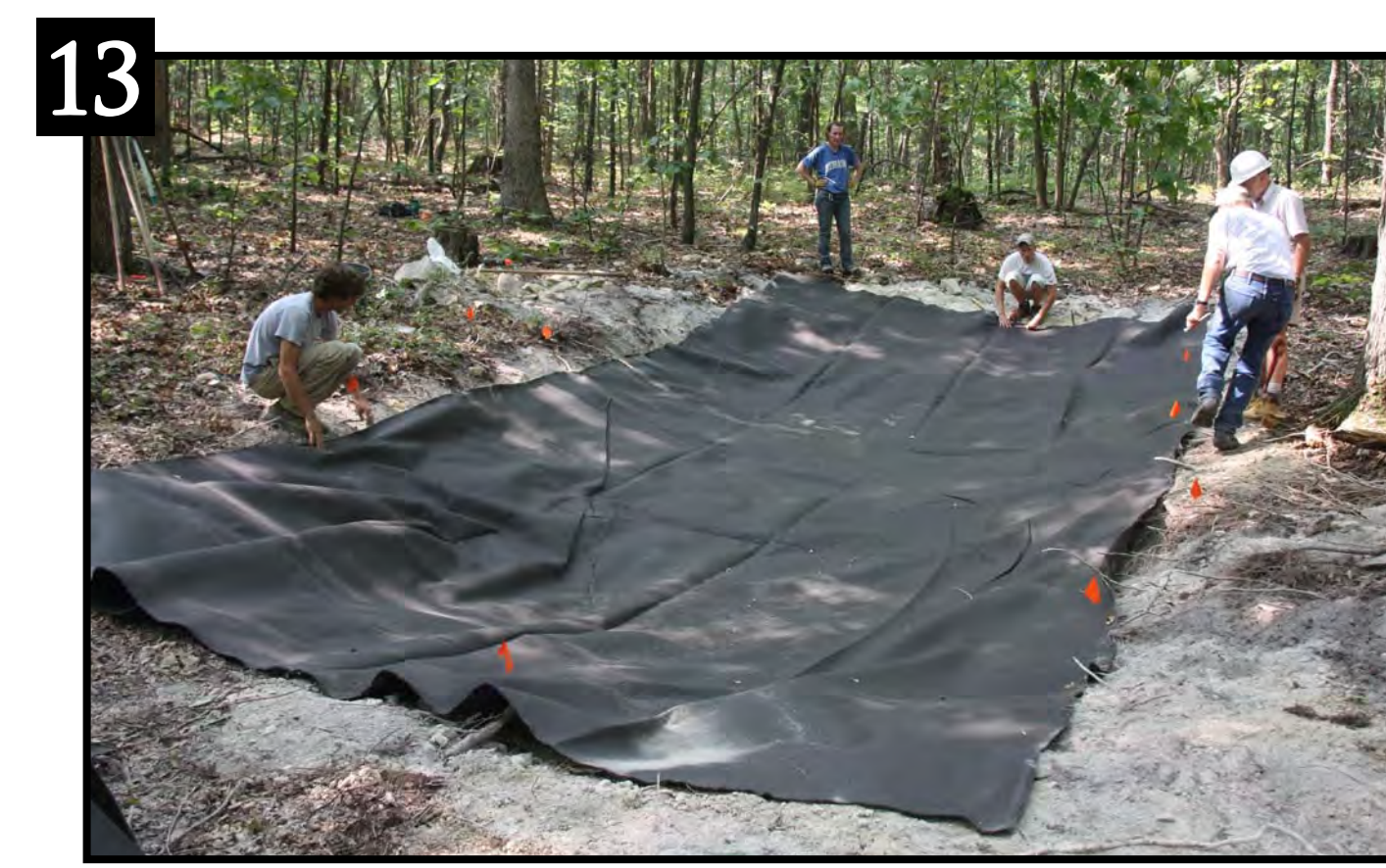
13 The orange flagging marked the high water-mark of the pool and indicated placement of the liner and pads.
