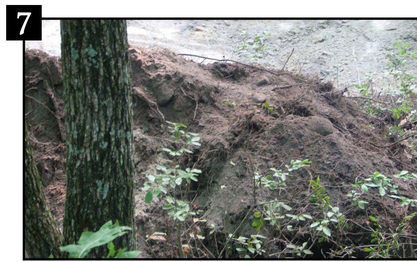
7 Topsoil was set aside for replacement after construction.
