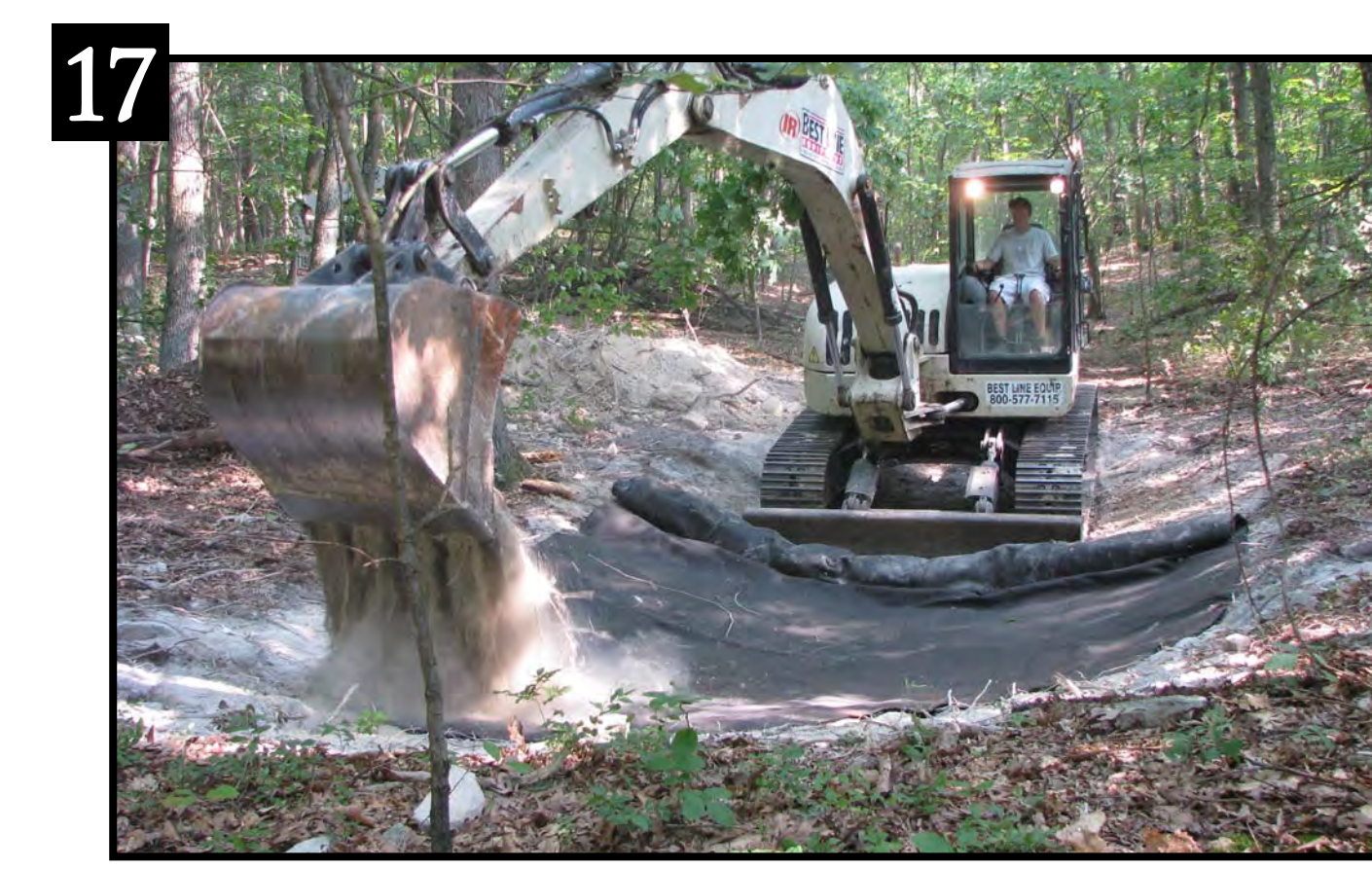
17 Rolling the liner allowed the excavator to drive closer to the secured half to replace soil.
