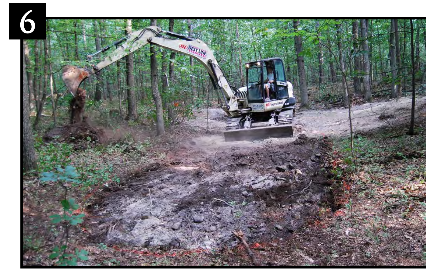
6 The basin dimensions were marked and topsoil was removed using the excavator.
