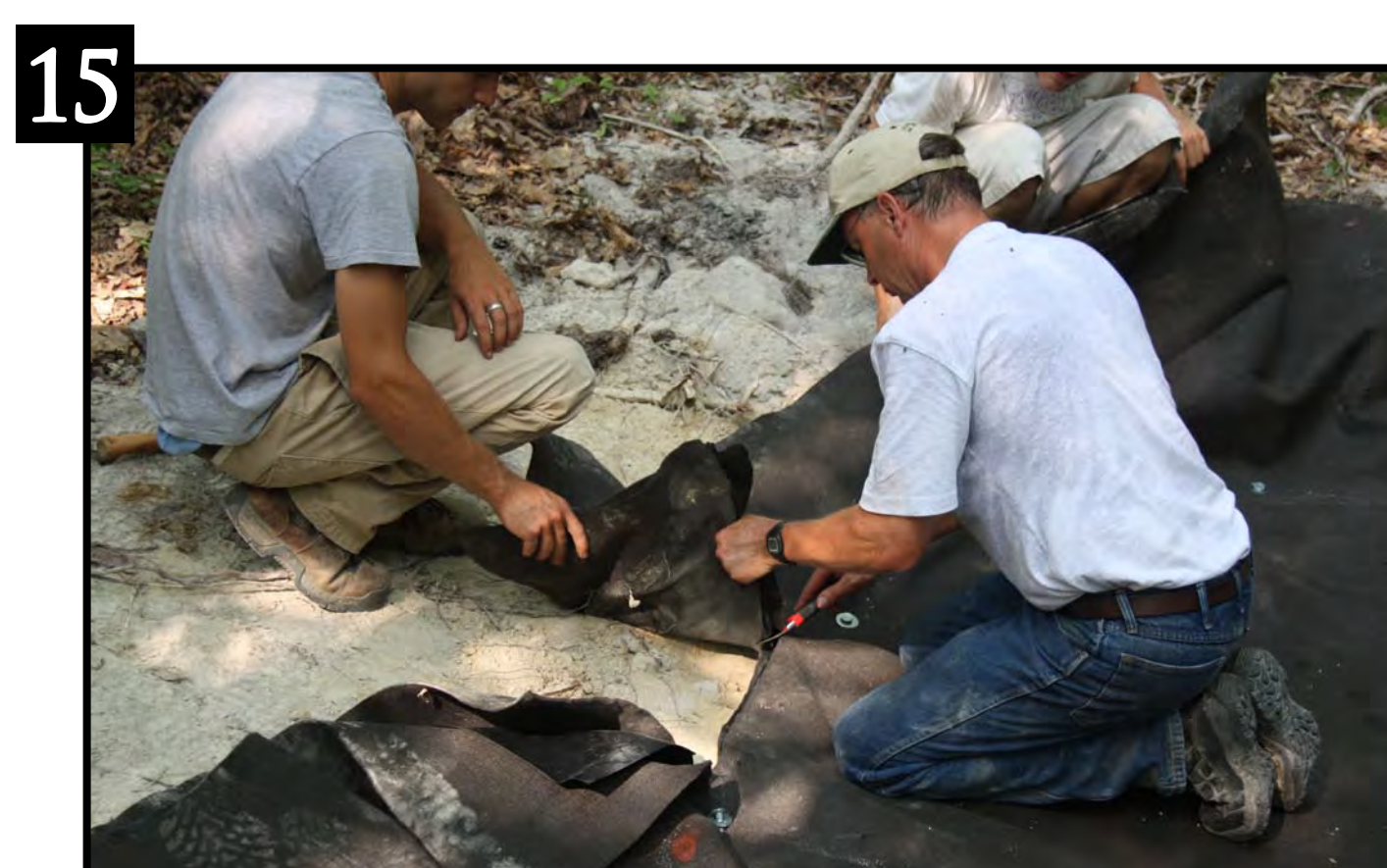
15 Once the liner was secured, excess material was trimmed from above the spikes.
