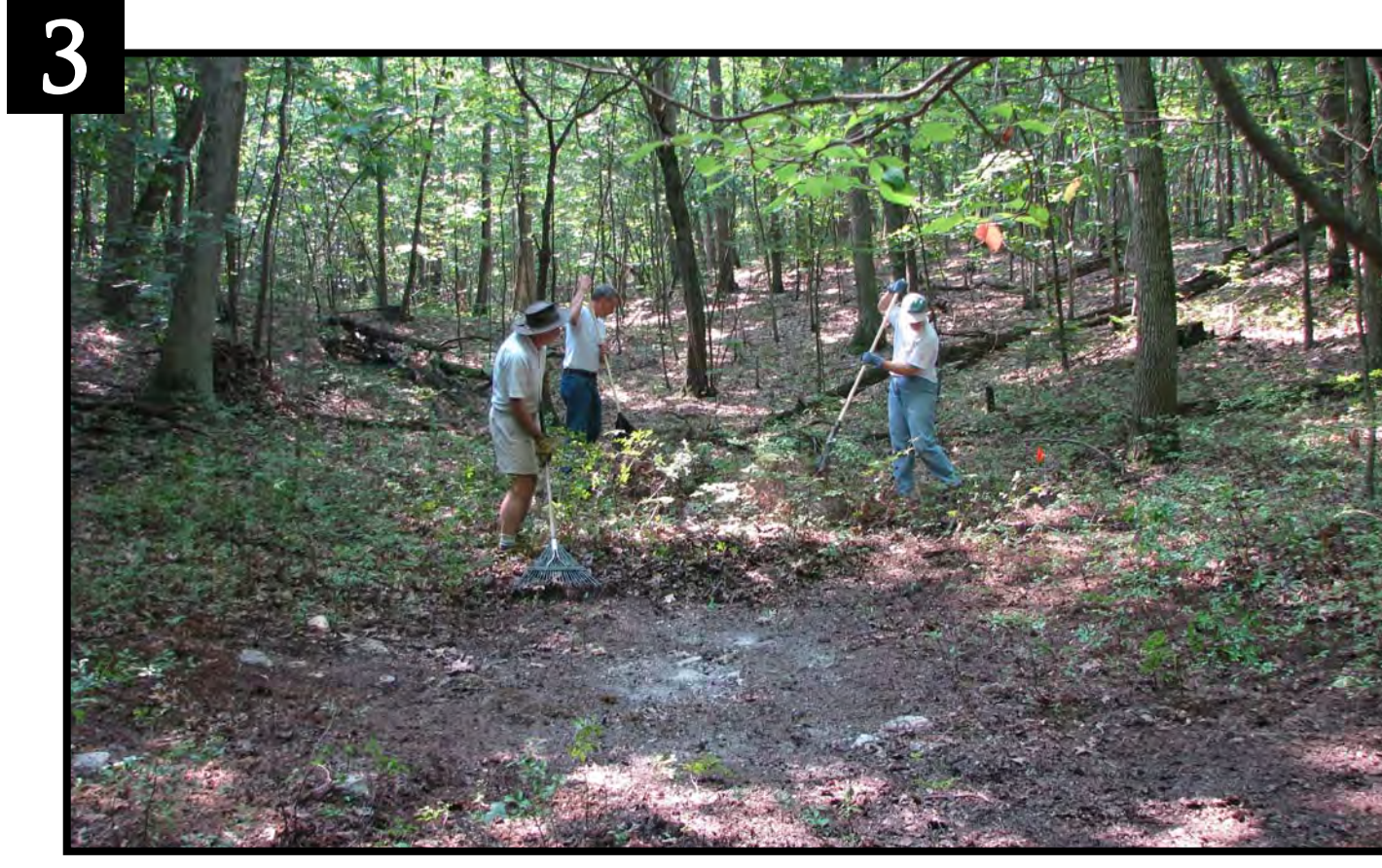
3 Leaves were raked from the basin prior to construction and reserved.
