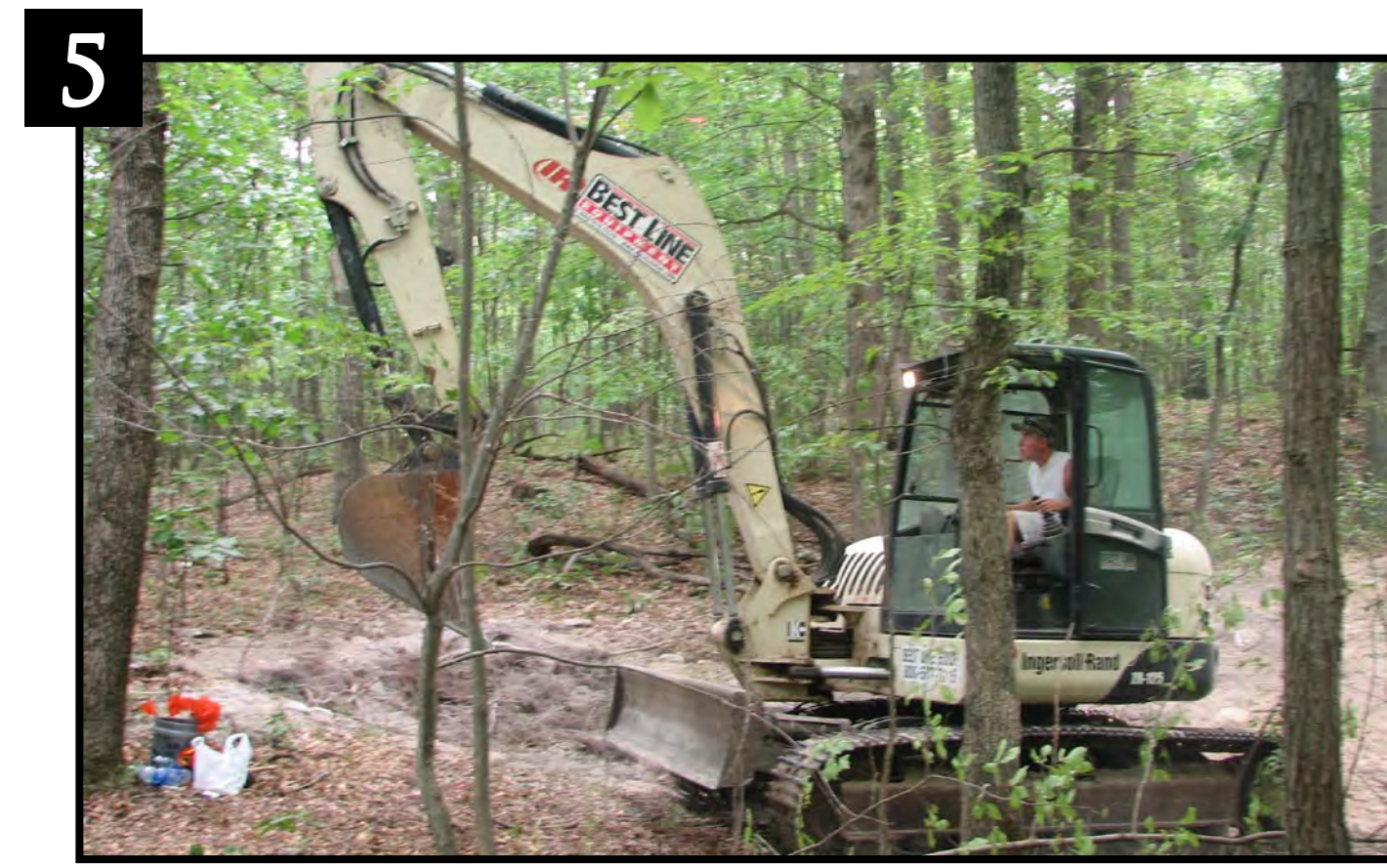
5 Predetermined access routes and careful navigation through the woodland minimizes disturbance to the construction site.
