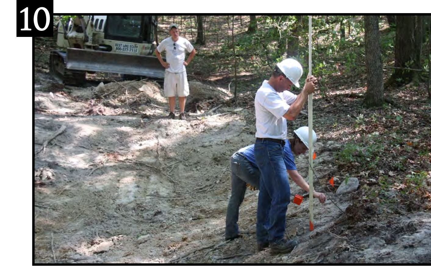
10 Target basin dimensions were marked and checked using the construction level and flagging.
