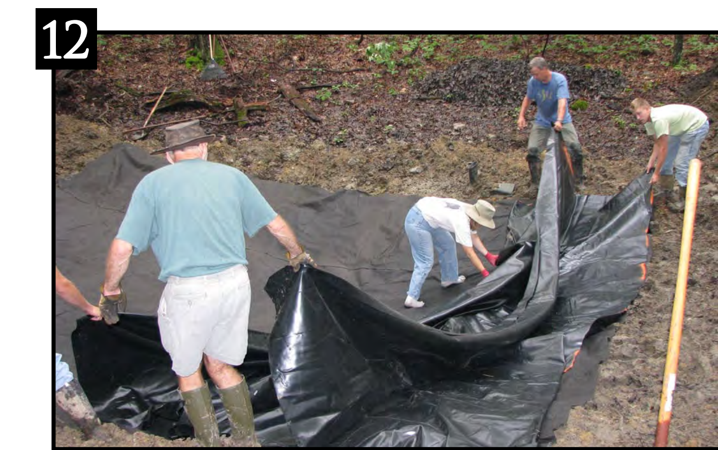
12 The three liner layers were placed in the depression one at a time. The 30 mil aquatic-safe liner was protected on both sides by 16-ounce geo-textile pads.
