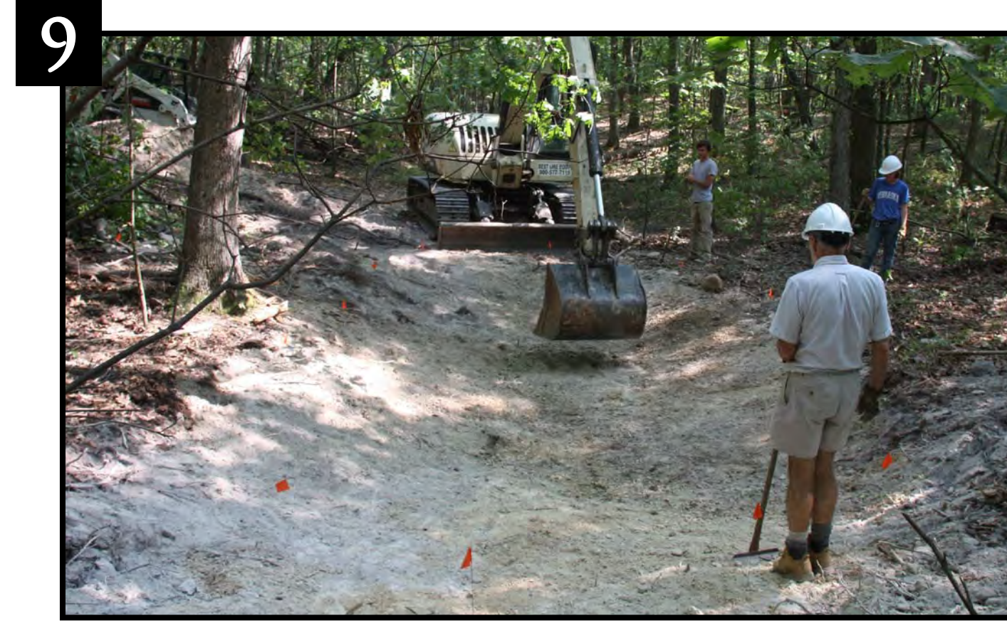
9 About 8 to 12 inches of mineral soil and rock were removed and set aside. A gradually sloped depression was shaped and compacted by the excavator.
