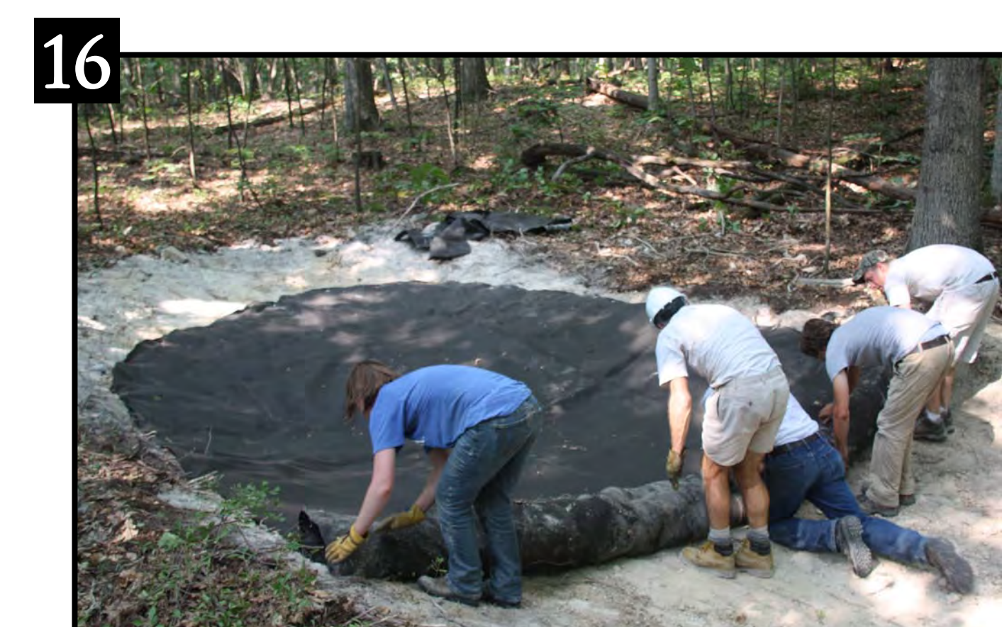
16 One half of the liner was secured, the other half rolled back.
