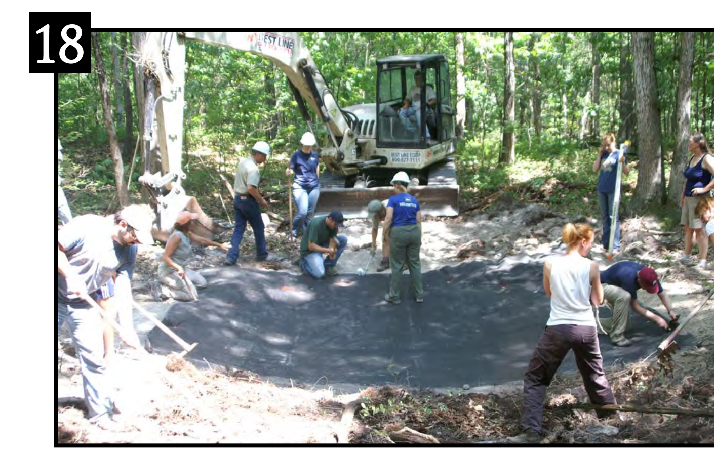
18 The second half of the liner was unrolled, secured, and covered with soil. Never allow machinery to touch or drive on the liner.
