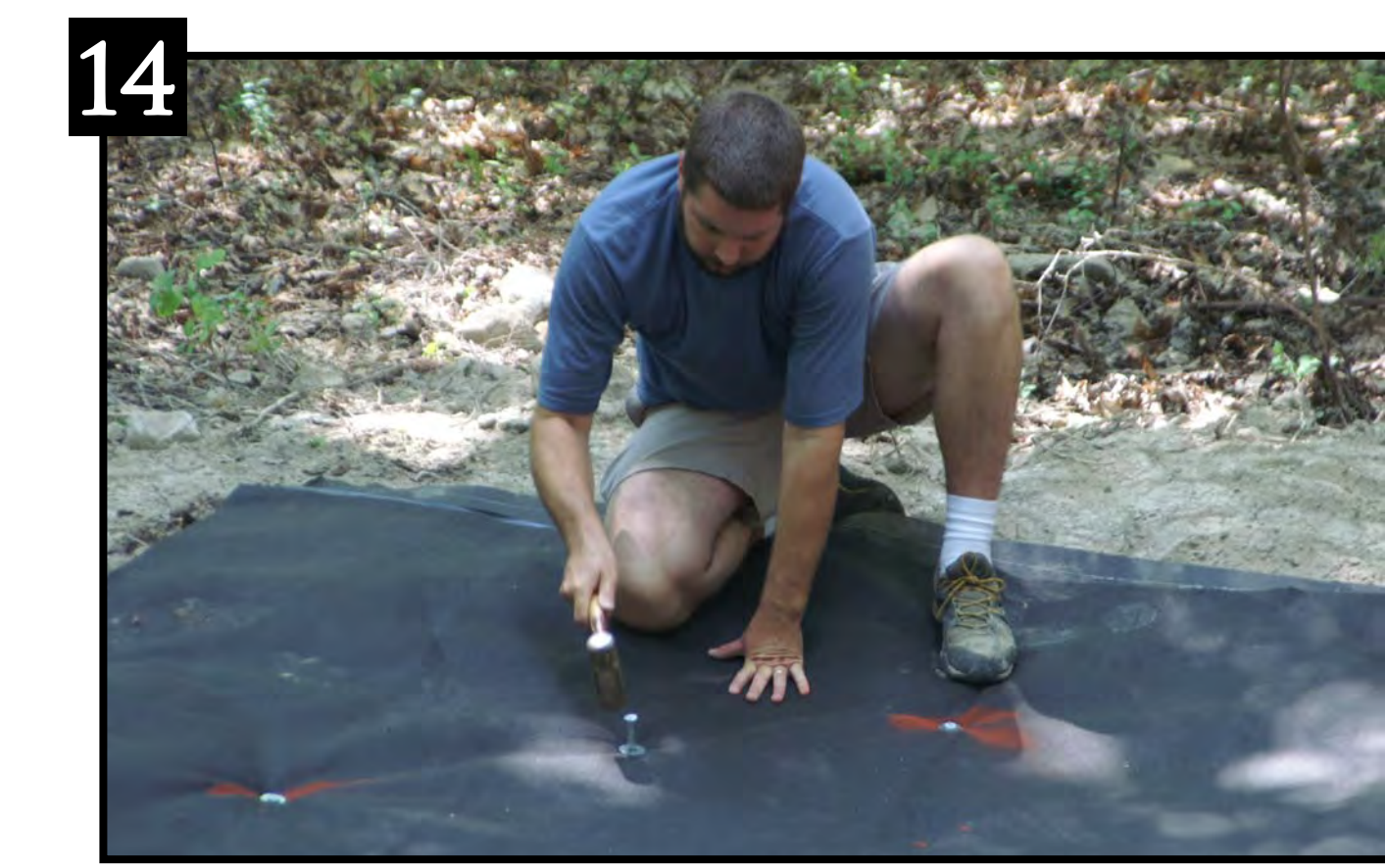
14 The three liner layers were held in place by 12-inch galvanized steel spikes and washers. These were placed along the upper edge of the liner at the high water-mark indicated with spray paint.
