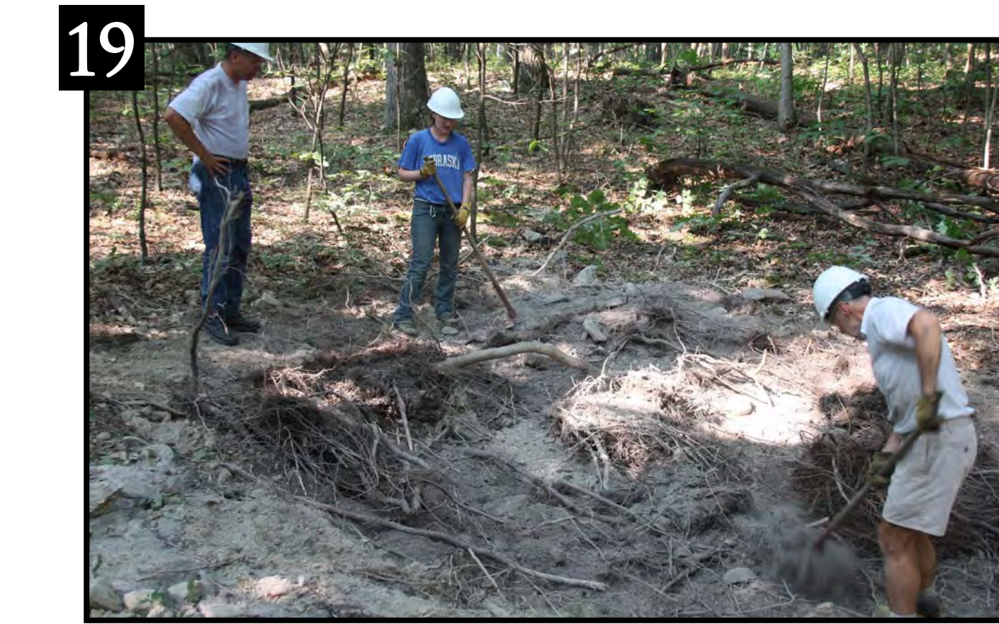
19 The mineral soil (photo 9) was replaced with 1 inch of topsoil (photo 7). Hand tools were used to smooth the upper edges of the basin.
