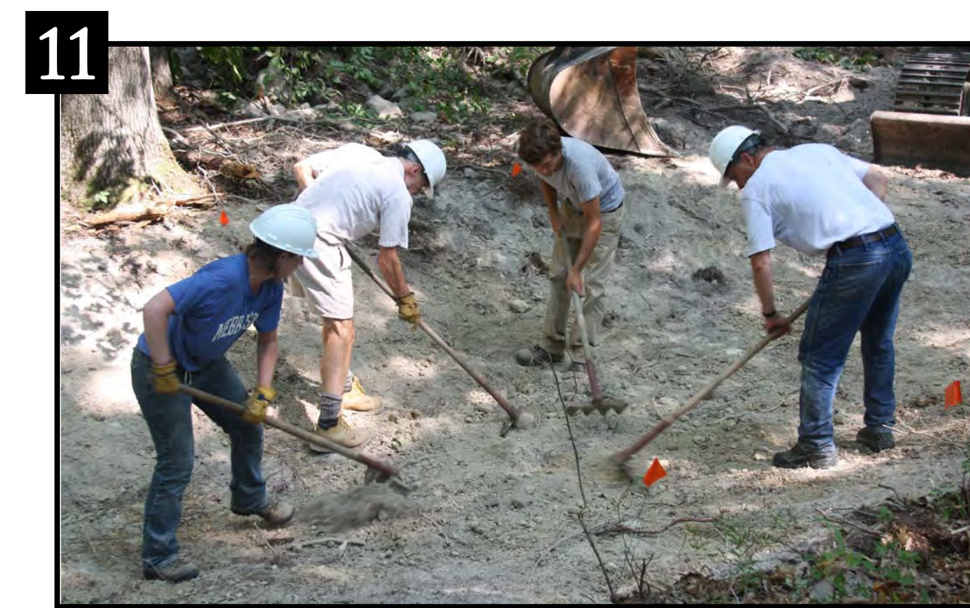
11 The rough excavated depression was smoothed by raking sideways and uphill. It was important to remove any sharp rocks or sticks from the depression to prevent puncturing of the liner.
