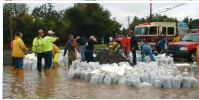
Preventing flooding in Hilton fire hall © MIKE LISSOW.
