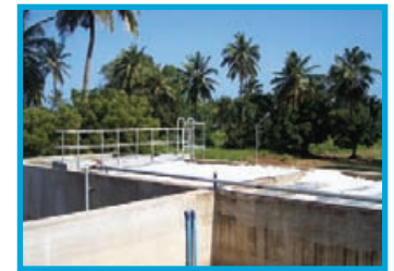
Our wastewater treatment requirement has initiated significant investment in facilities such as this one at a bottling facility in Kenya
