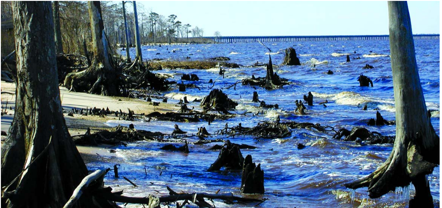
Exposed cypress roots and stumps along an eroded shoreline are a vivid sign of how sea-level rise and severe storm events are altering the Albemarle Peninsula's natural systems. ©Jennifer Henman
