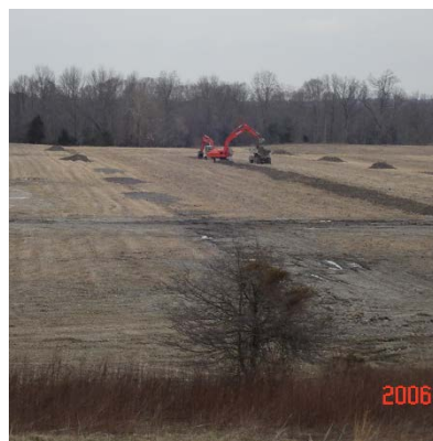
Filling field ditches in 2006.
