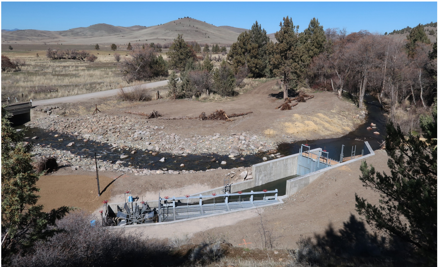
Figure 3. Aerial view of new diversion structure and reprofiled channel
