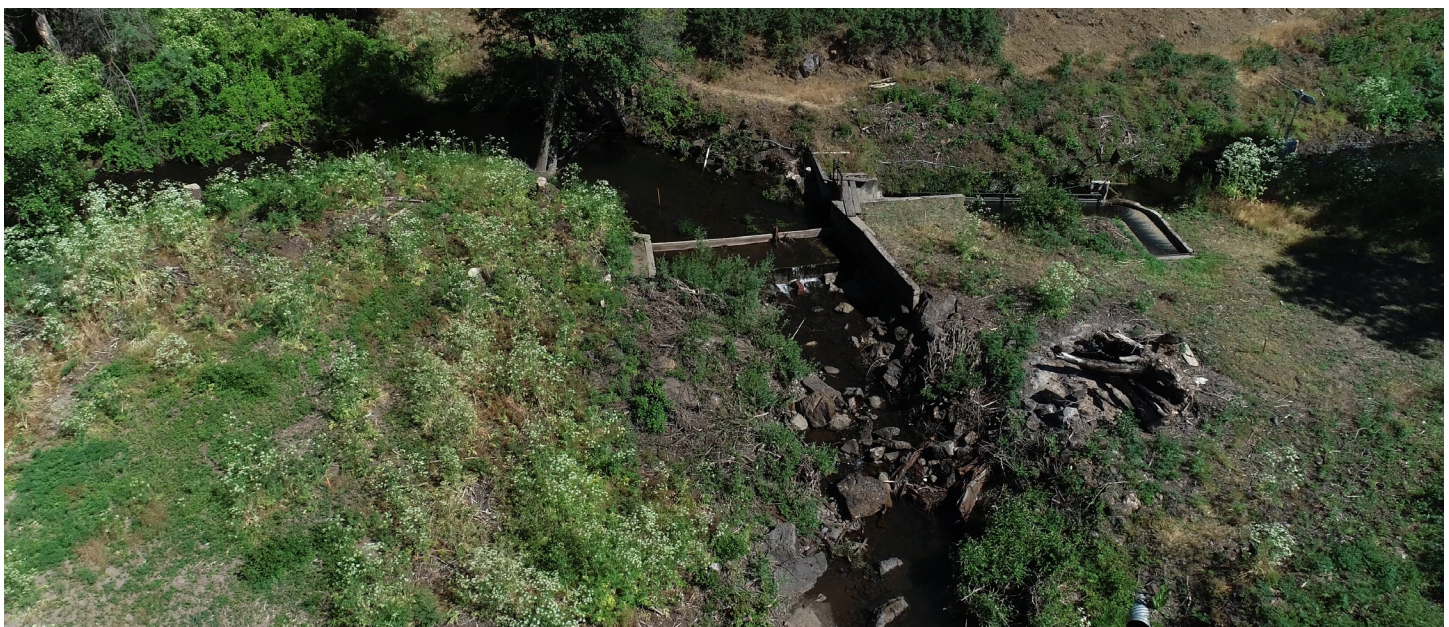
Figure 2. The old diversion structure that was a barrier to fish passage
