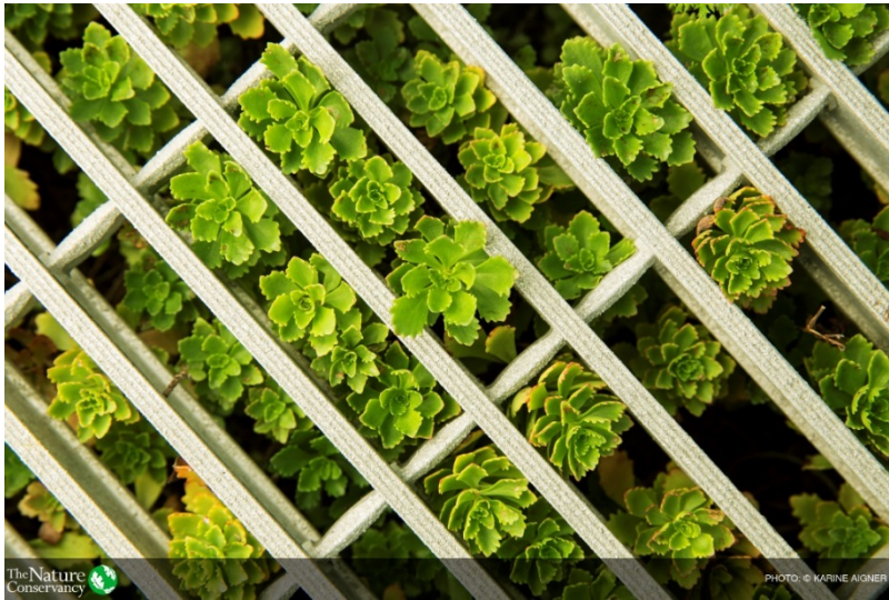
Green roof on the American Society of Landscape Architects in Washington, D.C.
