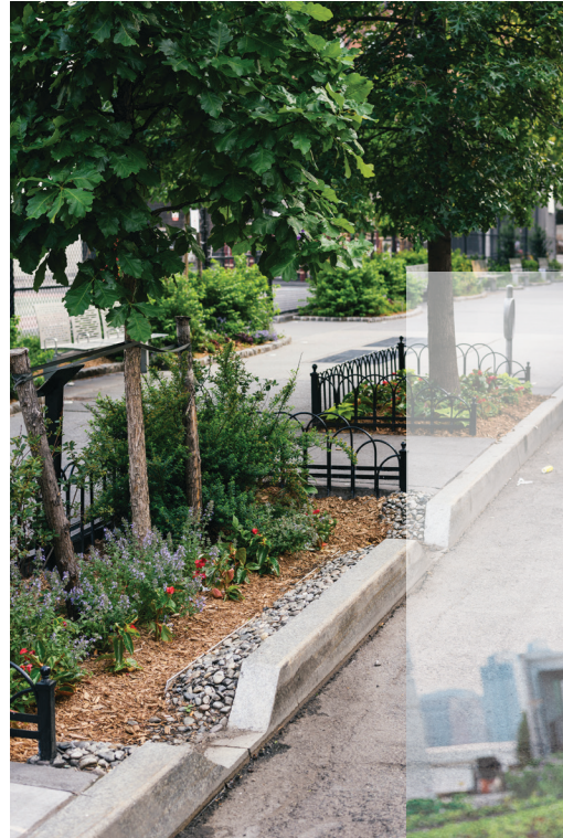
Working with neighborhoods to plan for more urban nature can help strengthen a community. A sidewalk bioswale (above), like this one in New York City, can clean stormwater runoff, reducing pollution in rivers and bays. Harvesting greens at the Brooklyn Grange Rooftop Farm, which grows more than 50,000 pounds of organically cultivated produce per year.
